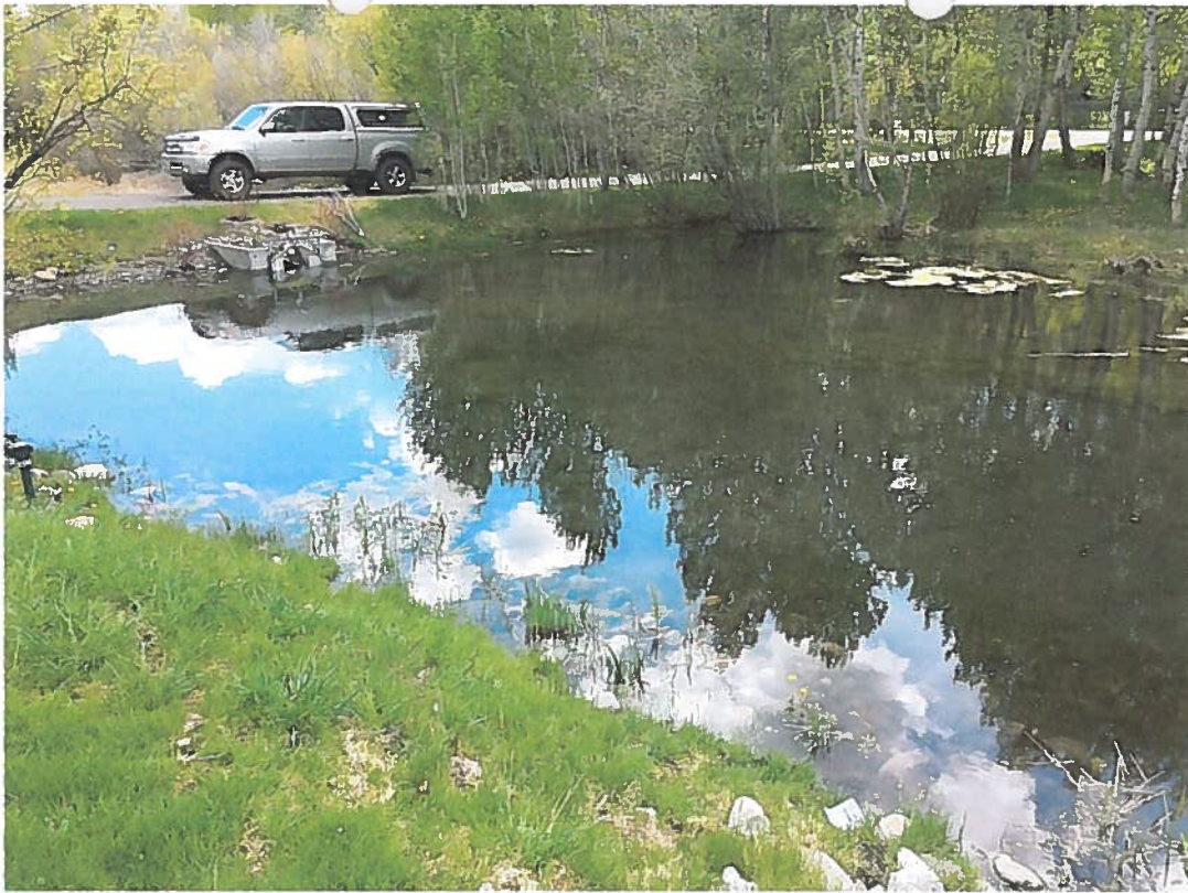
Lower end of pond showing check / measurement device
