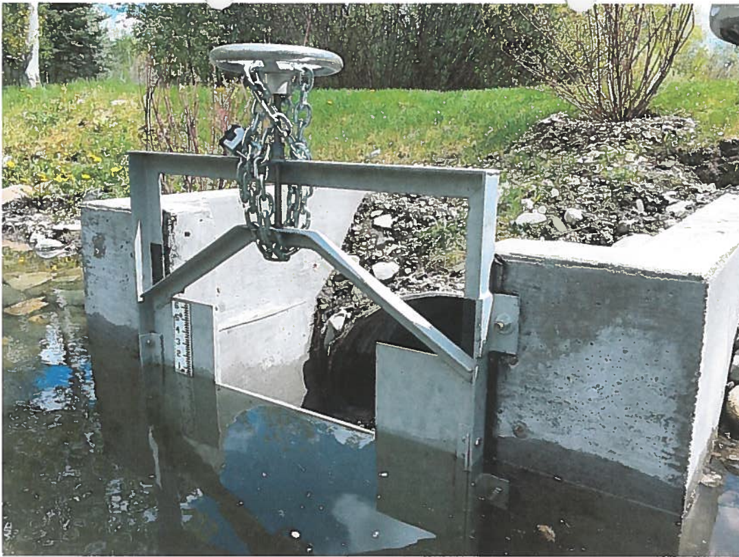
Outlet structure and flow measurement weir
