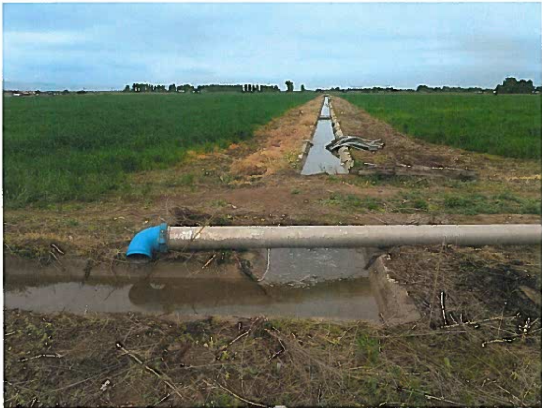
Figure 5: Looking west at the 8-inch pipe that discharges into the southern gravity ditch. Surface water can also be delivered into the gravity ditches from the New York Irrigation District as is occurring in this photo.
