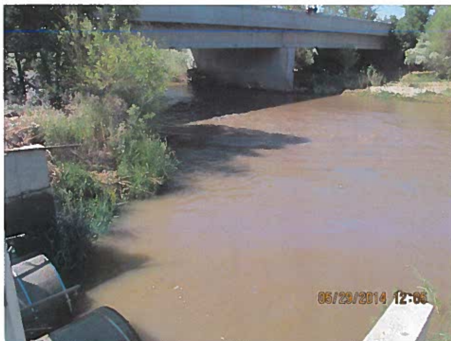
Bridge crossing Bruneau River upstream of pumping station. Pump intakes on left.
