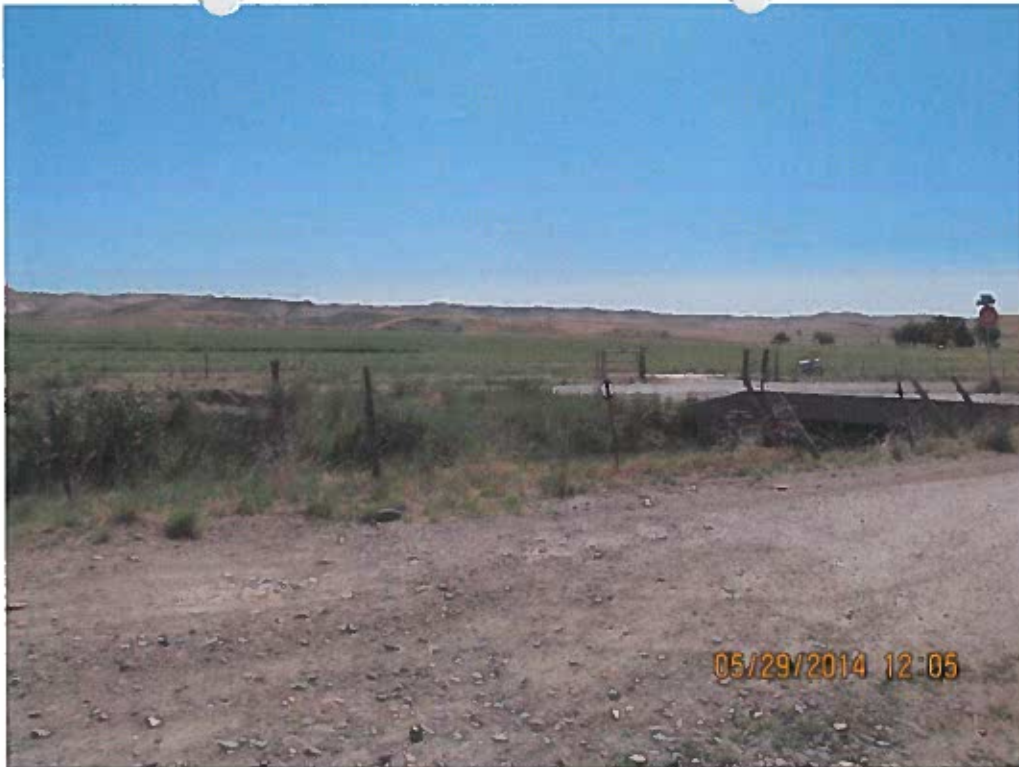
Looking east from pumping station across Bruneau-Buckaroo Ditch. These fields irrigated from 100 hp pump
