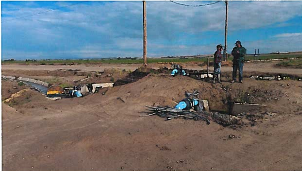
Figure 4: Three 8-inch open discharge points approximately 250 feet west of the well. Siphon tubes are used to draw water from the concrete delivery ditches once the water has been discharged from the well into the ditches.
