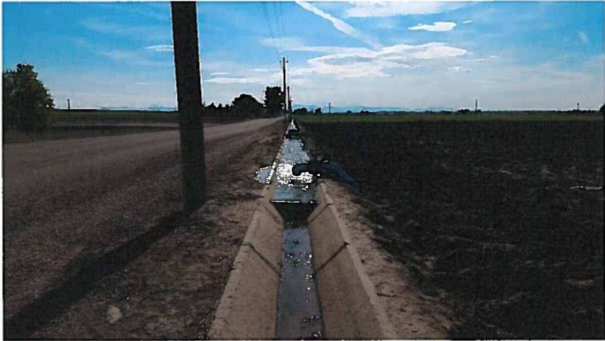
Figure 5: One 8-inch open discharge point approximately 50 feet east of the well.
