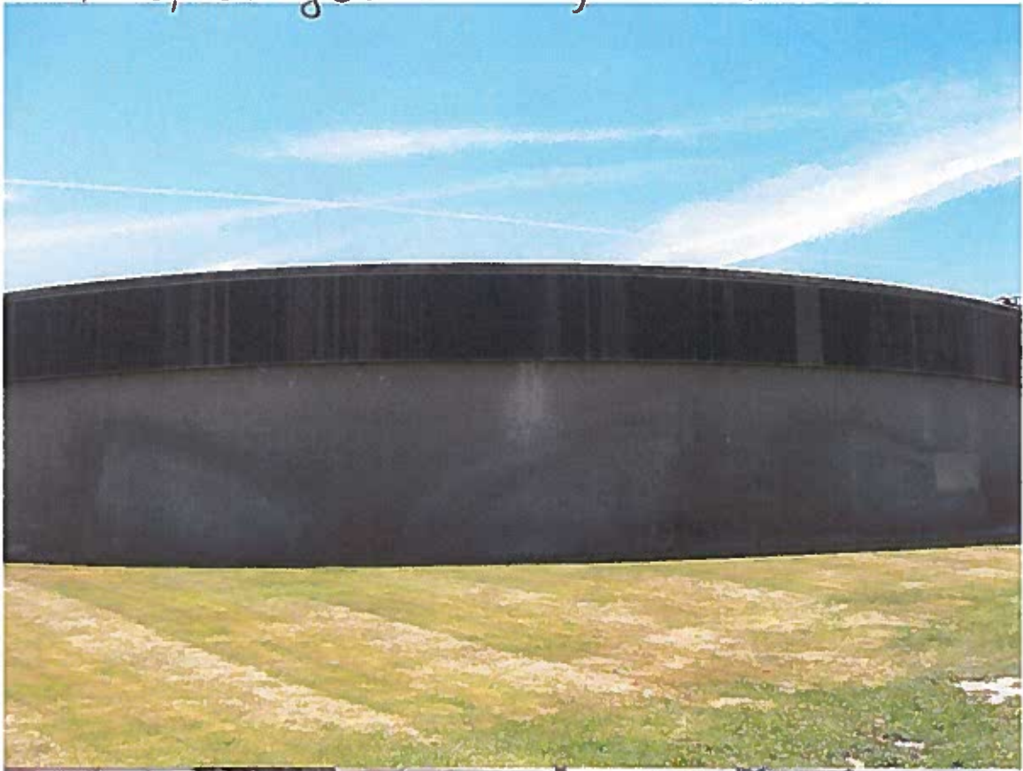
3,000,000 gallon storage tank
