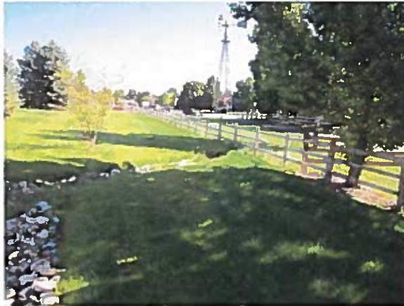
Overflow from Irrigation Pond
