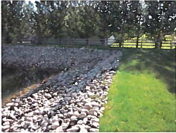
Burm by Irrigation Pond
