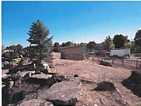
Recirculation pump house
