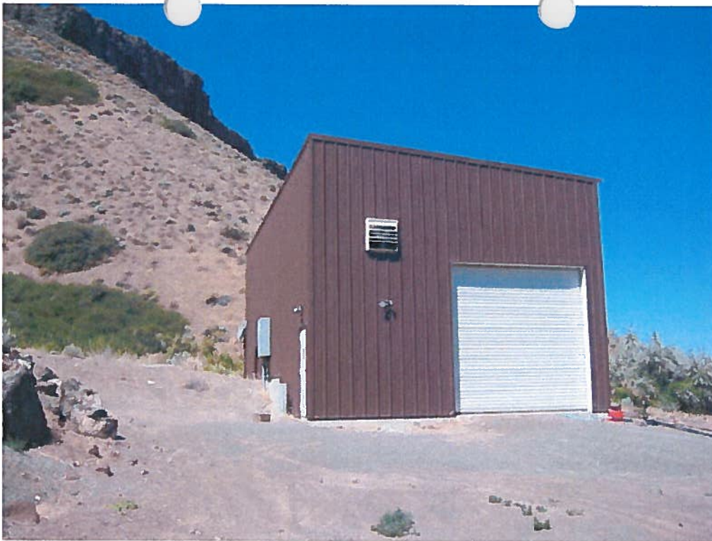
Power house in Snake River Canyon
