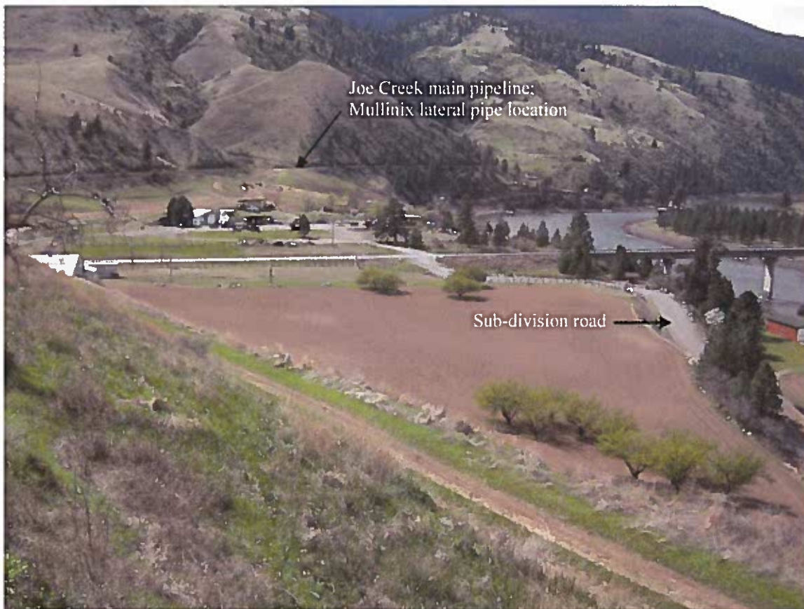
Figure 12 View of lower Killgore irrigated field in foreground; Mullinix irrigated field visible in far background just below old Joe Creek ditch cut or grade where mainline is now buried.
