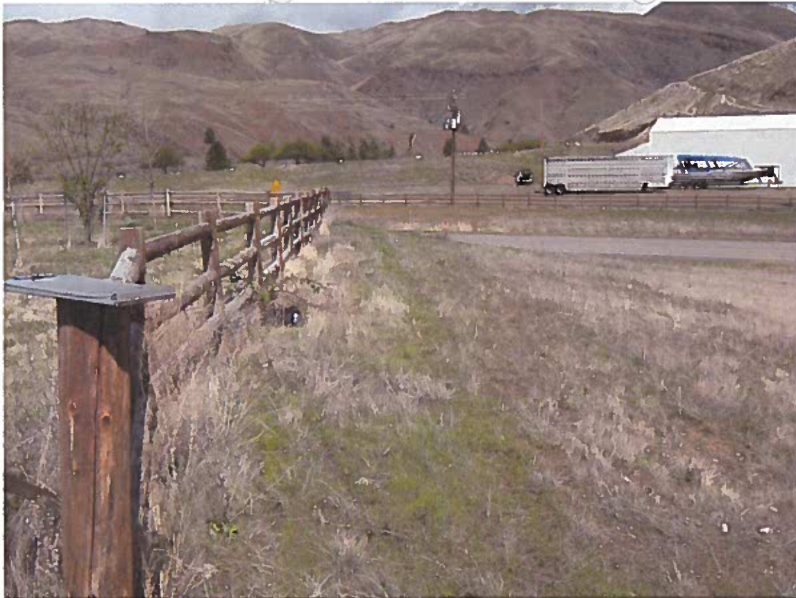
Figure 9 K Killgore fence line and Highway 95 (middle of photo). Buried mainline pipe is along fence line and to right, then crosses highway. Killgore/horseshoe bend property or area is on other side of highway.
