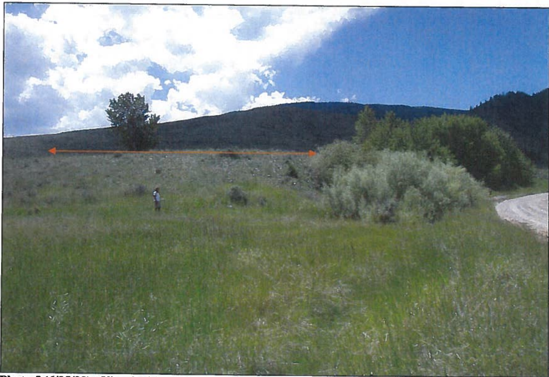
Photo 5 (6/25/09) - View looking at the downstream slope of the dam near maximum section. Note the location of Oliver Road (right), and the heavy growth of vegetation on north side of the embankment.
