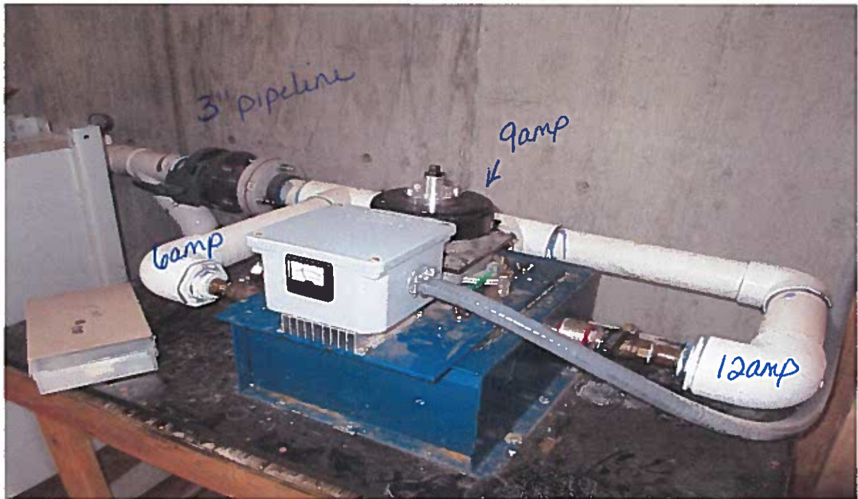
Generator with 3-way switch change flow based on need. Return flow is on the back of blue box Harley Generator
