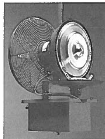
Pictured above is IVI's Centrifugal Humidifier ceiling mounted with 2-blade fan and fan guard option.
