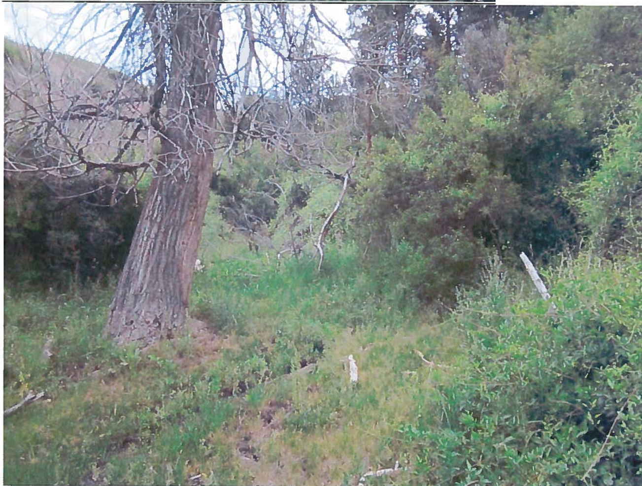
Pipe at the bottom of the ravine
