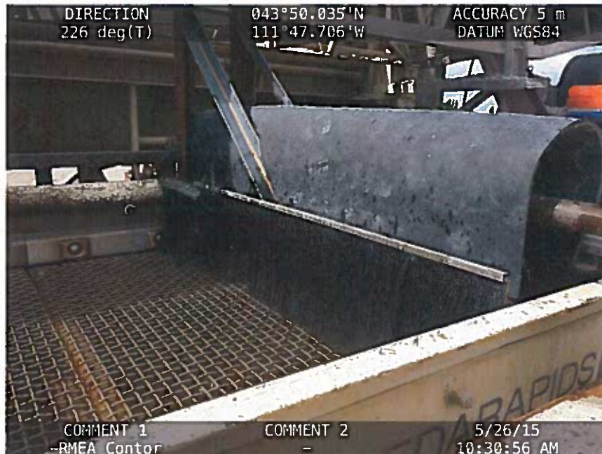
Photo IMG_0624.JPG. Belting and brushes used to shield sprays on lower screener. Photo taken with sprays operational.
