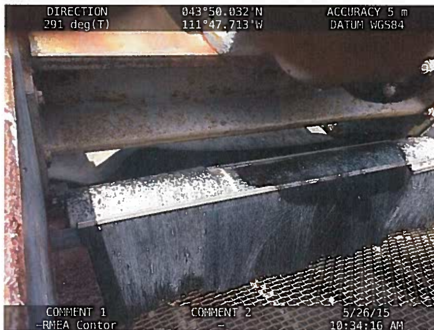
Photo IMG_0631.JPG. Brushes used to prevent lateral entry of wind into spray area of upper screener. Spray was operational when photo was taken.
