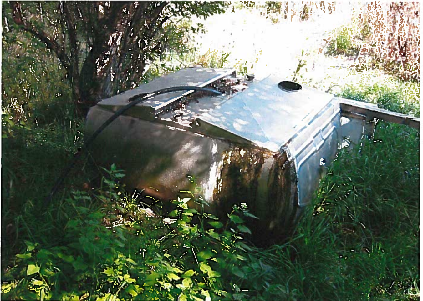
Hose runs into box at pool
