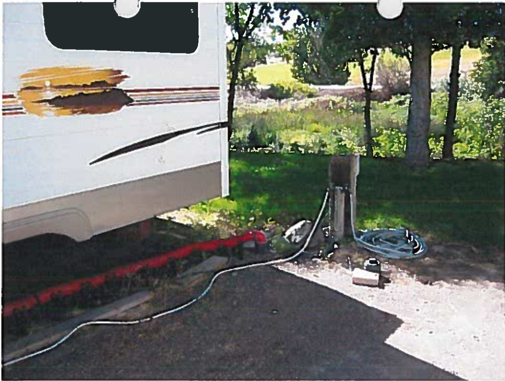
Water Faucet at Trailer Park at the Clear Lake Country Club
