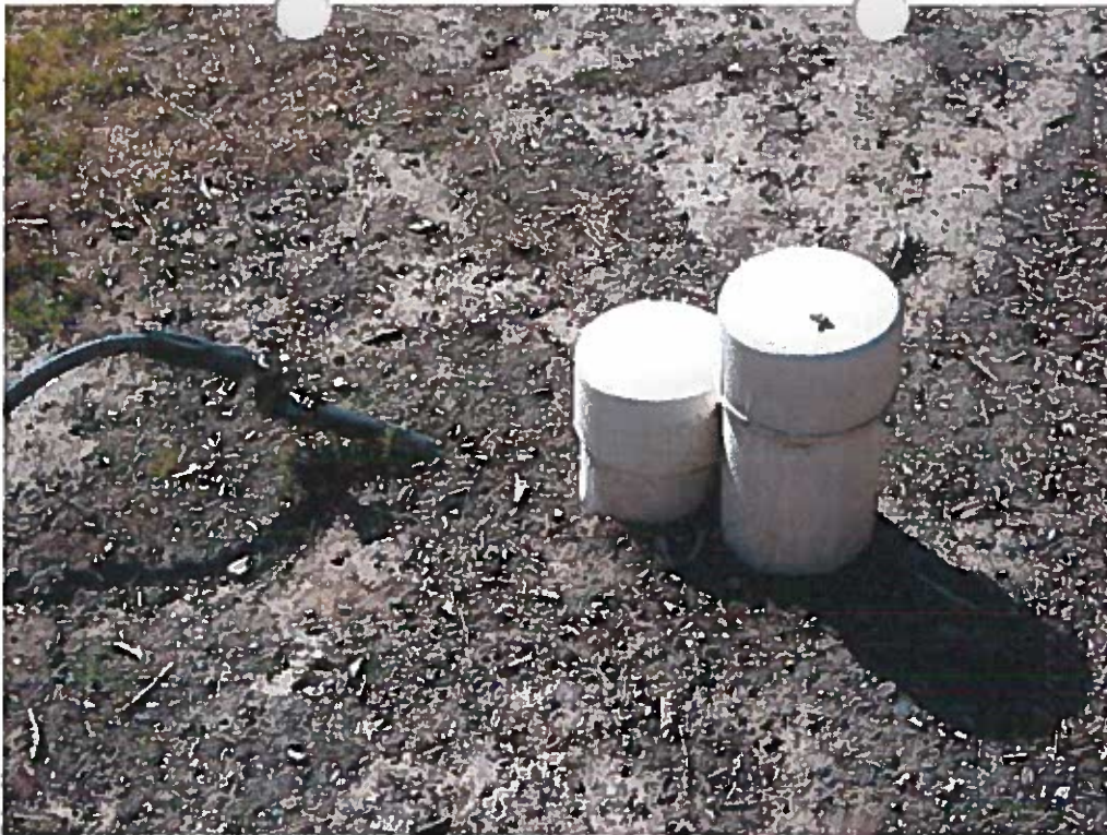
Stub-out at Empty Lot
