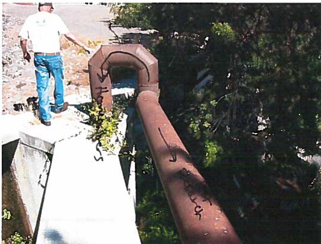
B. Twelve Inch Delivery Pipe After Leaving Point of Diversion
