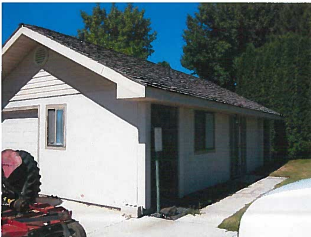
D. Pump House
