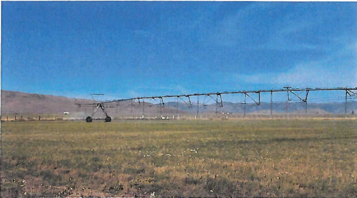
Response Photo 5 – North pivot and end gun operating
