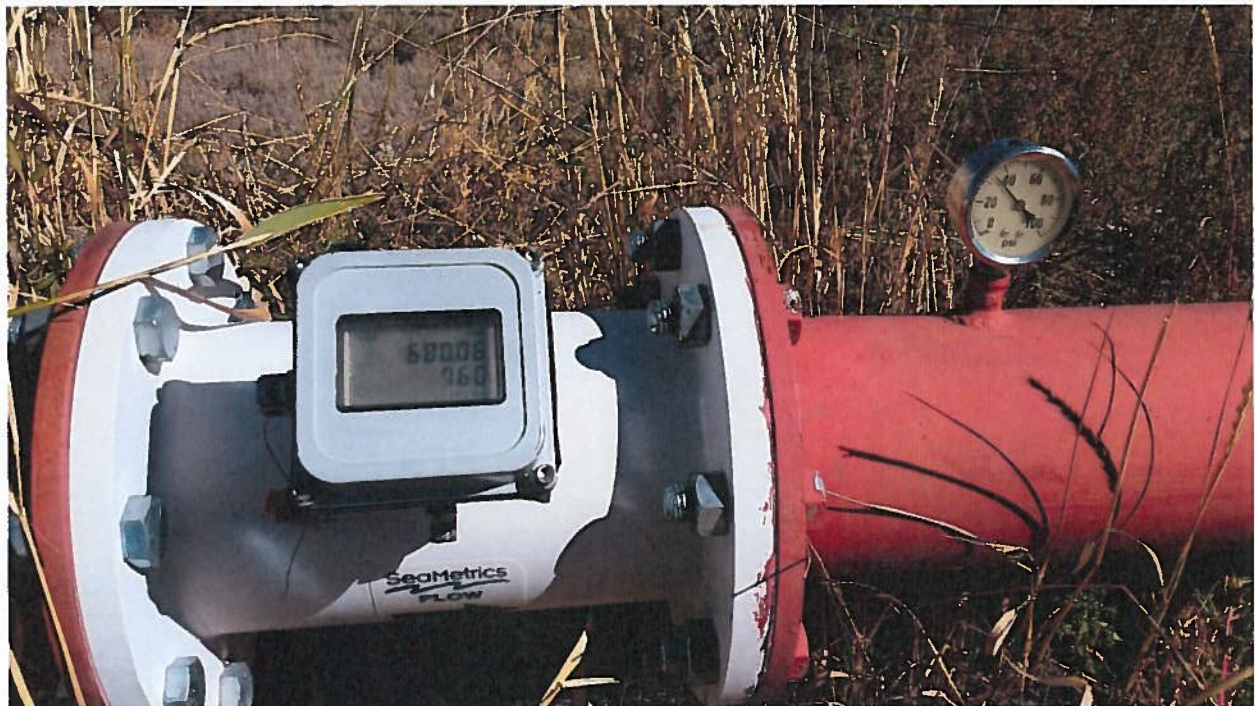
Response Photo 6: Flow Meter (680.06 acre-feet/760 gpm) and pressure gage (34 psi) during operation of 2 pivots with end guns and hand lines – after walking around site during operation
