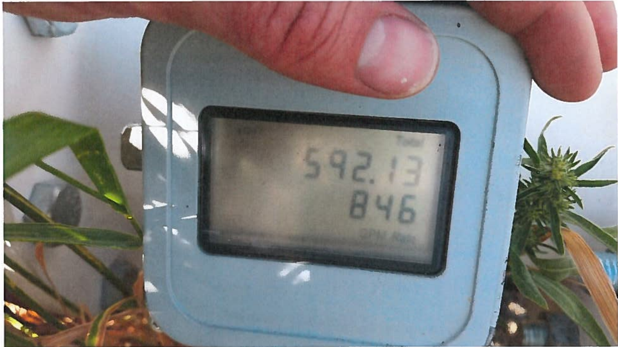
Photo 3: Photo of the installed Seametrics 6-inch flow meter on the well discharge pipeline. The Flowmeter read an instantaneous flow rate of 846 gpm, while the 10-minute averaged portable flow meter measurement computed to 837.7 gpm, a difference of less than 1%.
