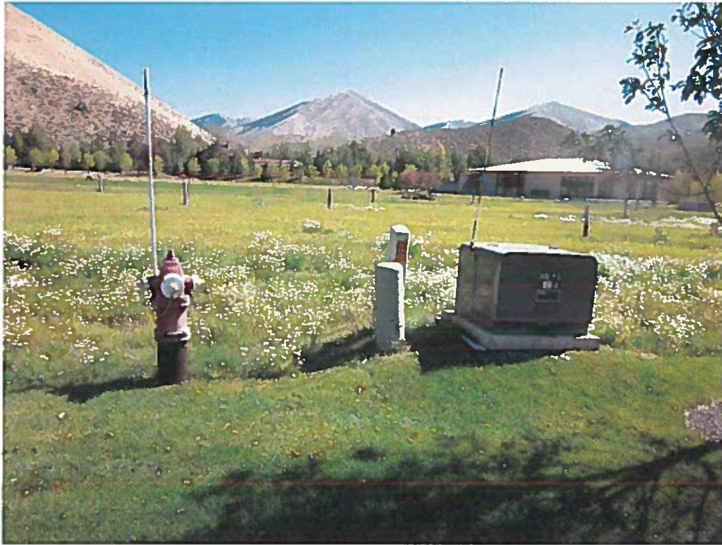
Figure 6: Power, telecommunications hookups and 1 of 7 fire hydrants
