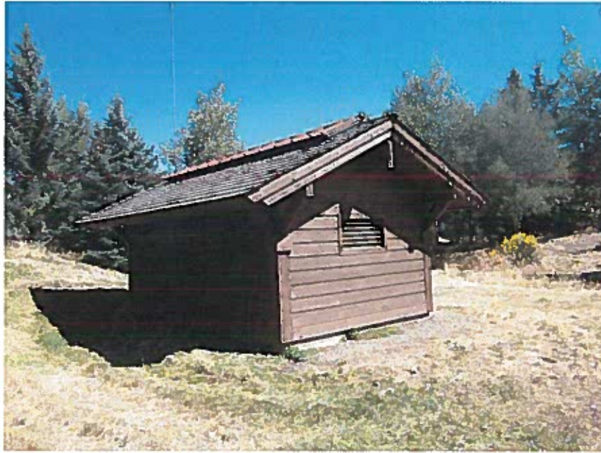
Figure 2: Pump House for Well #1
