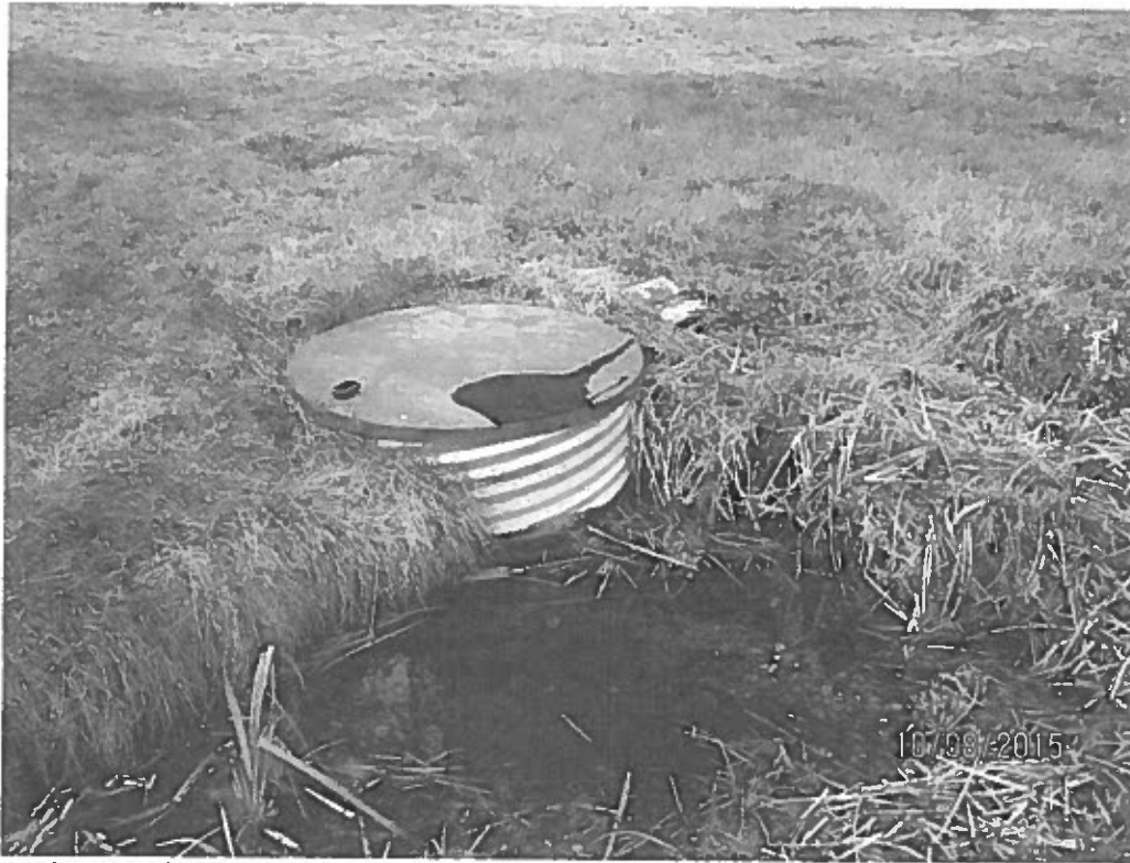
Photo 1: Picture of surface water diversion used for irrigation of lawn.
