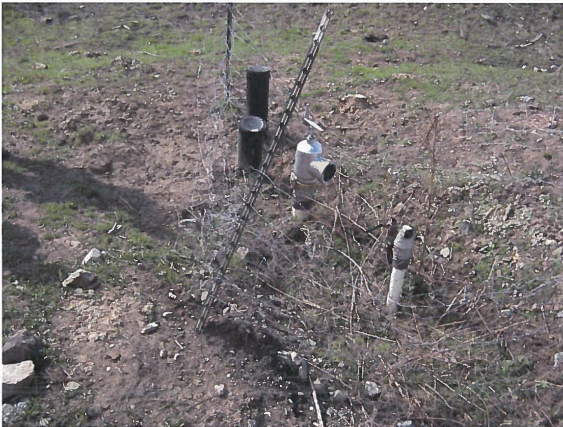
Figure 6 Mullinix buried 2 inch pipe from mainline with black plastic control valve pipe, riser connection and air vac.
