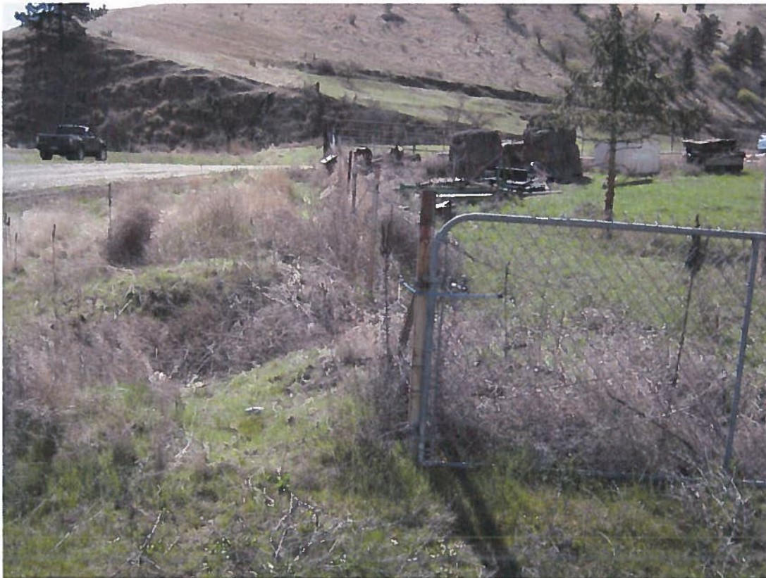
Figure 8 Location of buried mainline along fence lines (Karl Killgore's fence in foreground; Mullinix fence n background). Killgore hose bib/tap is behind metal gate/fence, in tumble weeds.
