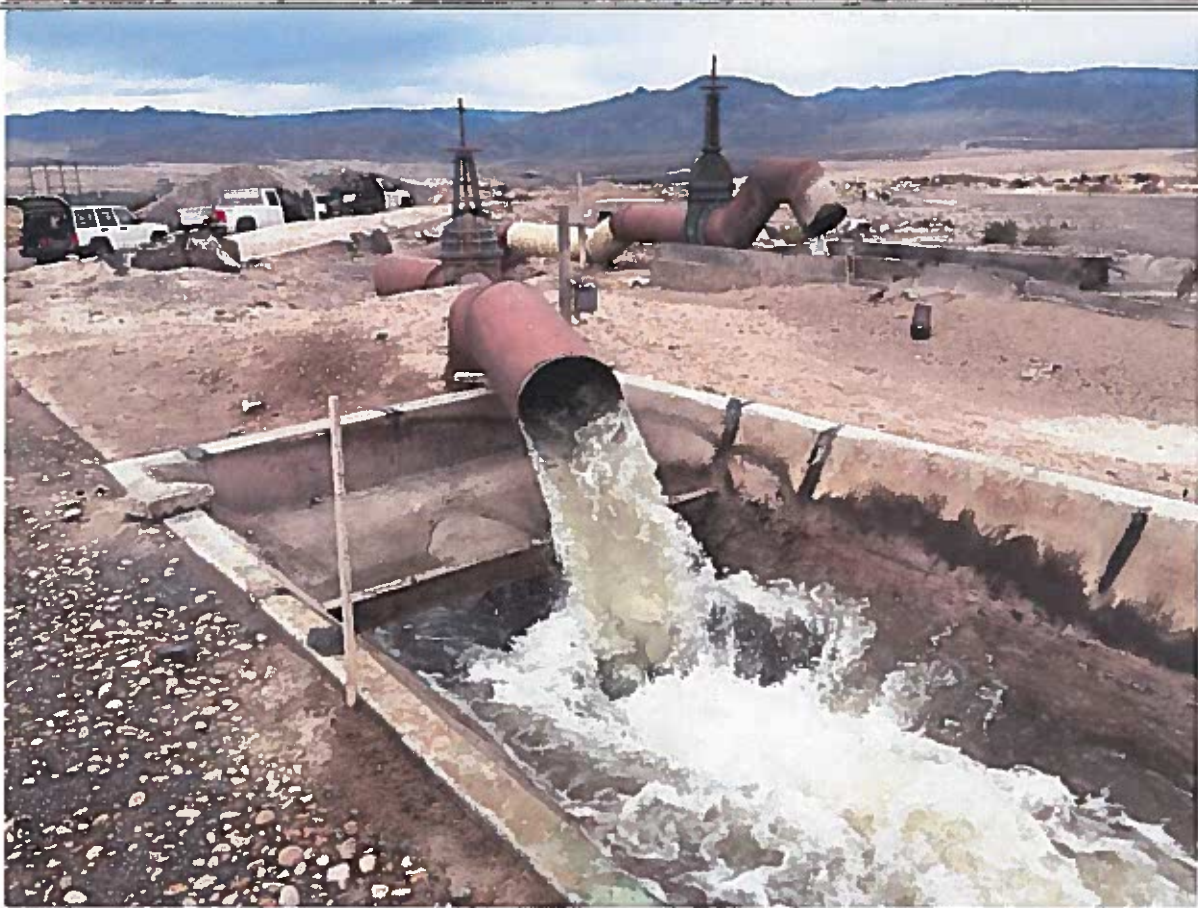
Snake River water is pumped into east ditch.
