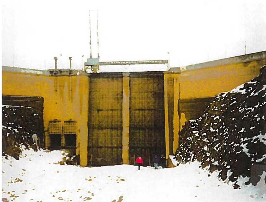
View of upstream end of powerhouse and powerhouse intake. Photo taken 12/09/96.
