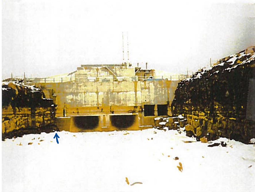
View of discharge area at downstream end of powerhouse.
