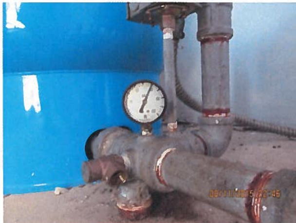
Pressure tank 60 PSI
