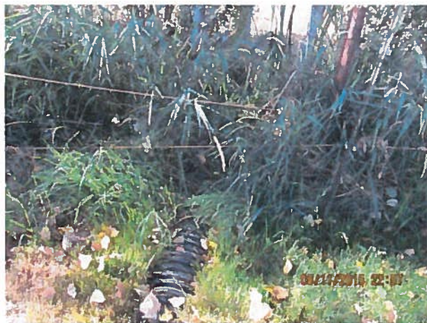
Discharge end of buried pipe located South of property
