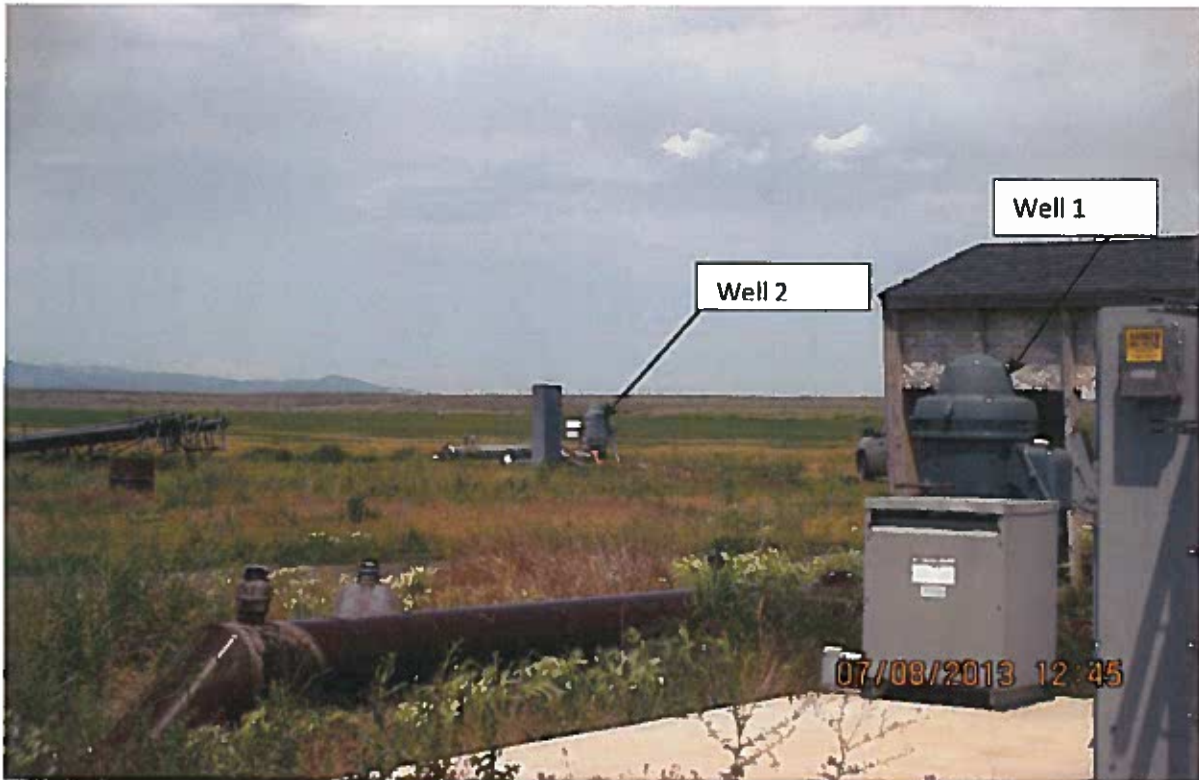
Well 1 & 2, 120 feet apart, facing Northwest
