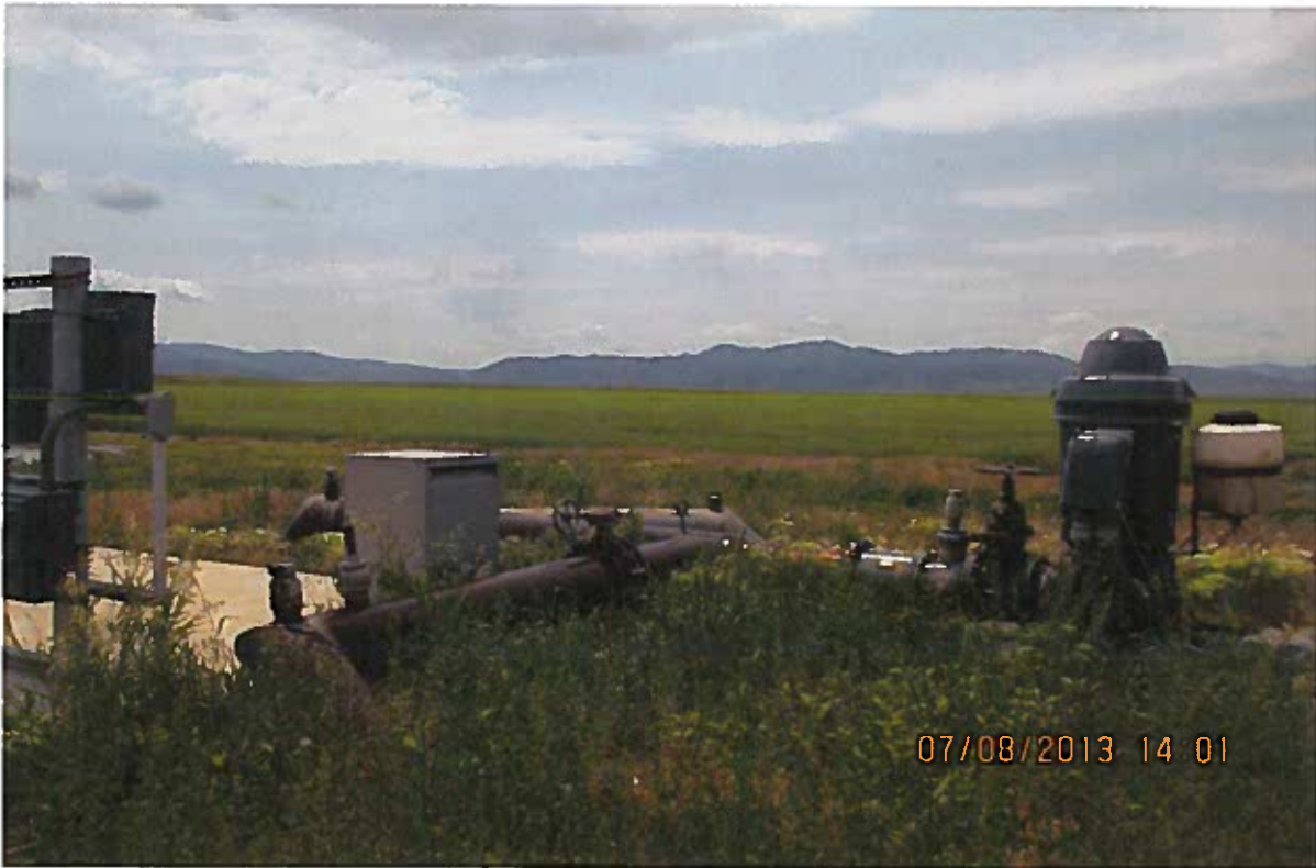
Well 1, Looking West
