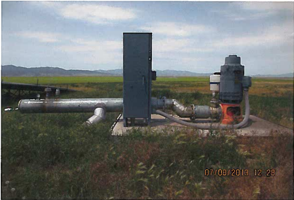
Well 2, looking West
