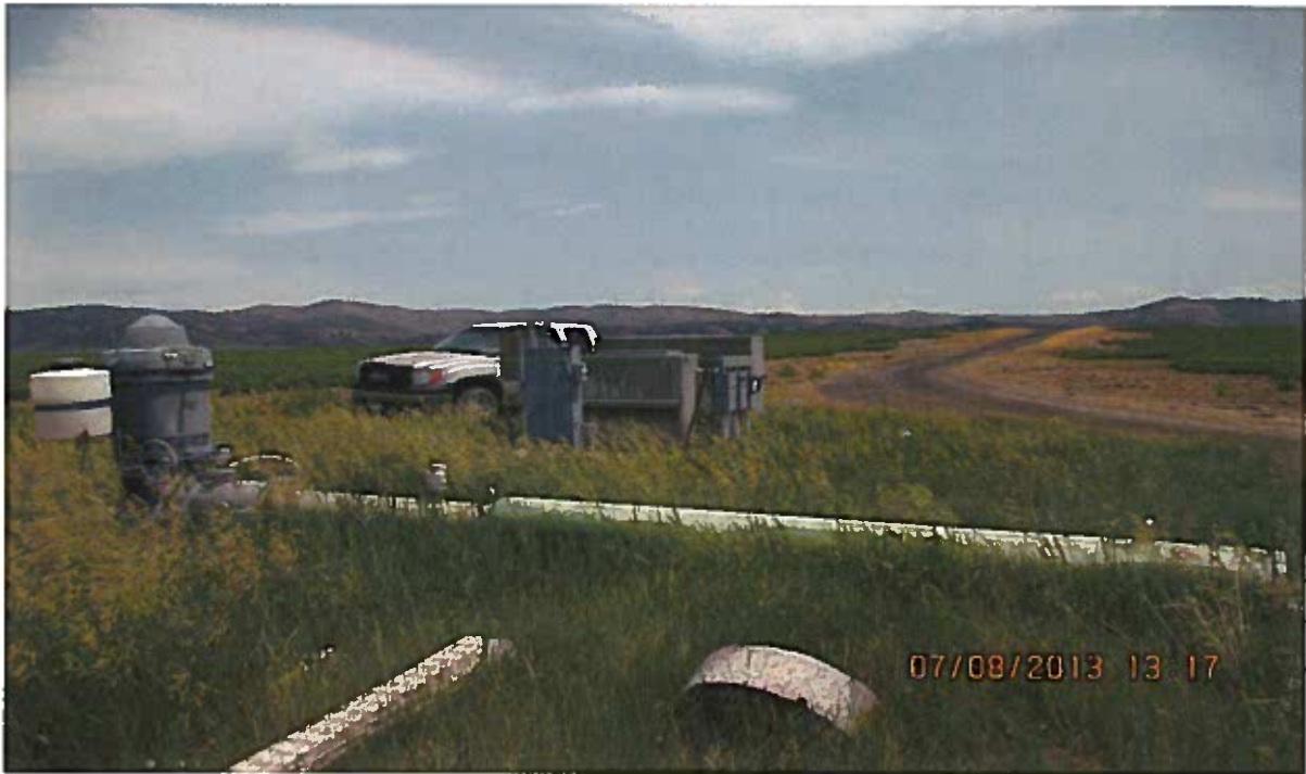
Well 3, looking West
