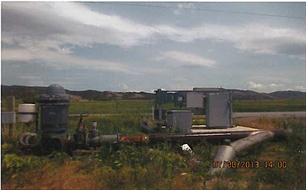
Well 1, looking East
