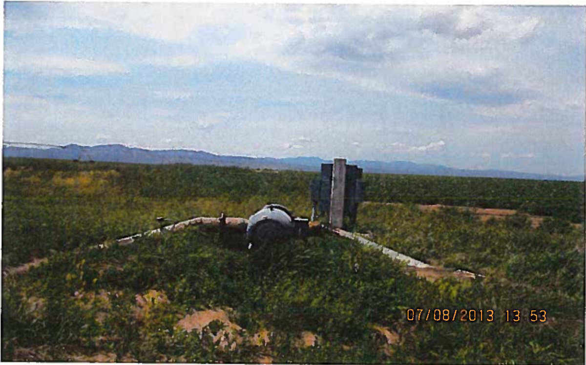
Booster Pump, looking West
