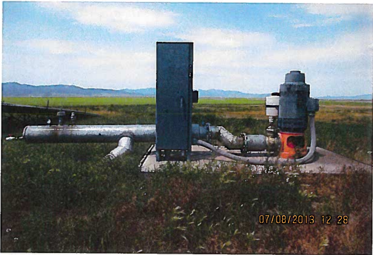
Well 2, looking West
