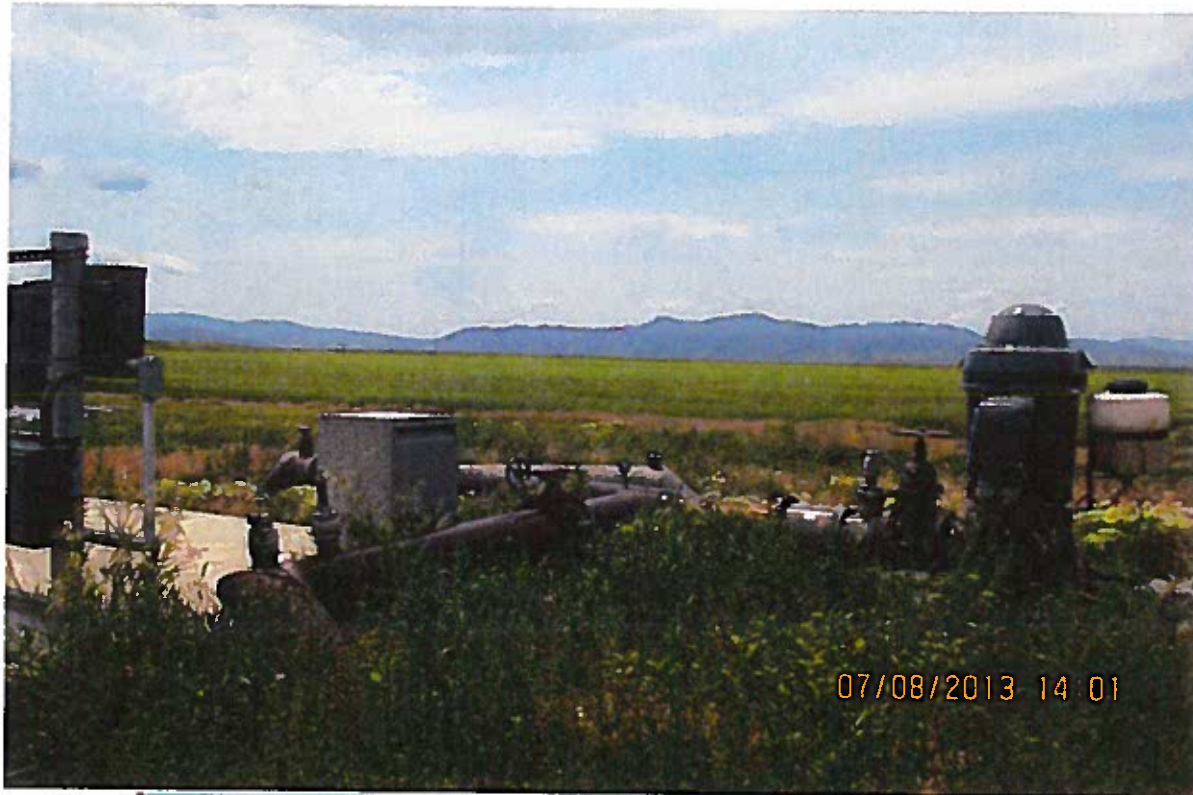
Well 1, Looking West
