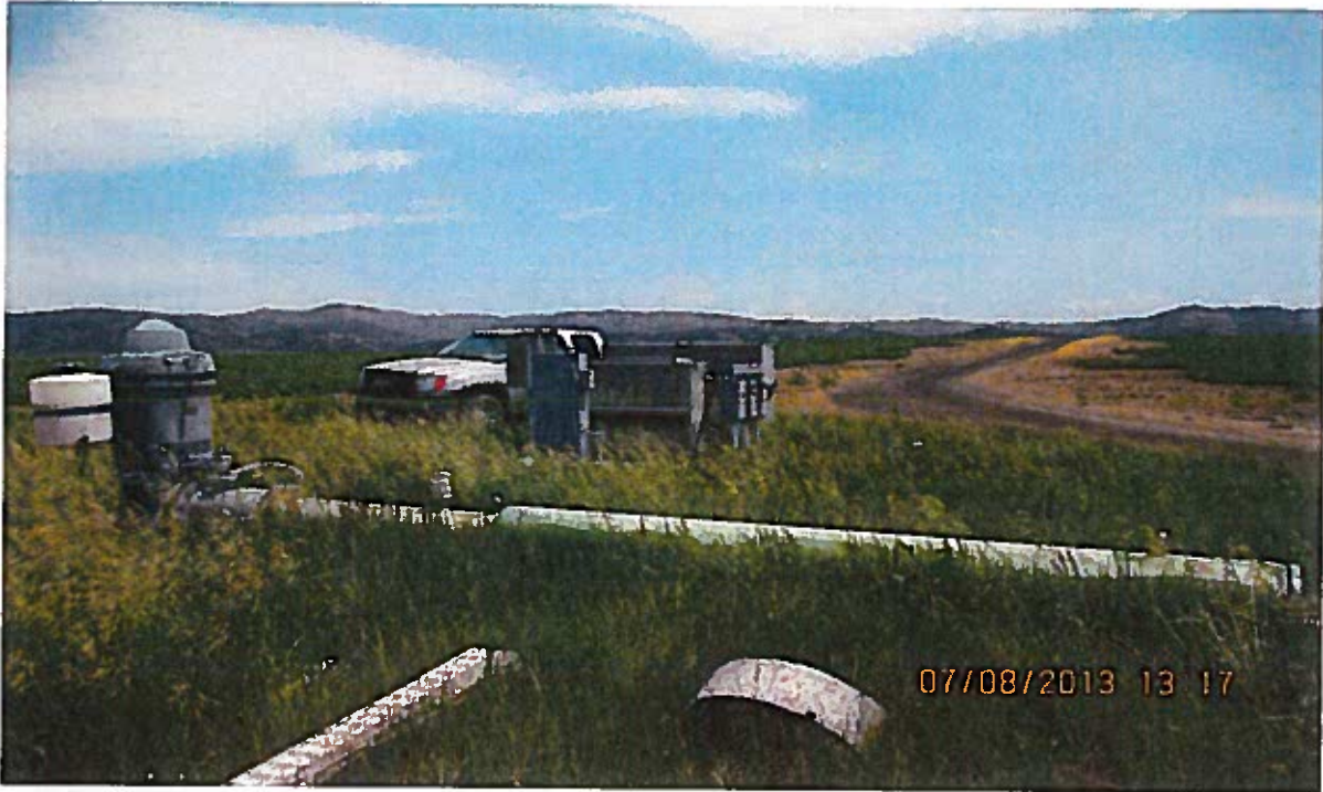
Well 3, looking West
