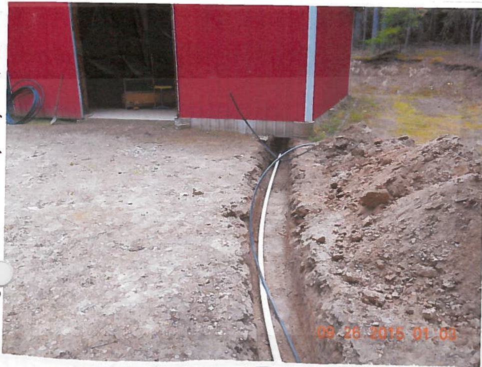
Water hooked to faucet, and power run to garage
