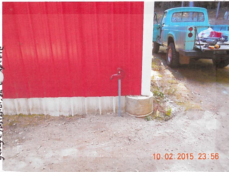
cabin installation complete
