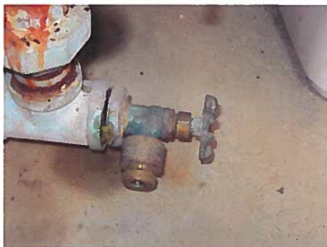
12. Corrected item from the previous survey.
