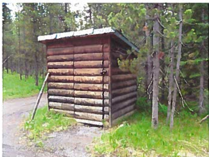
11. Pump house for the Back-up Well.
