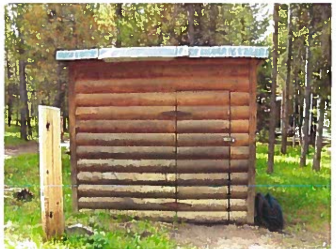
6. Pump house for the Main Well.
