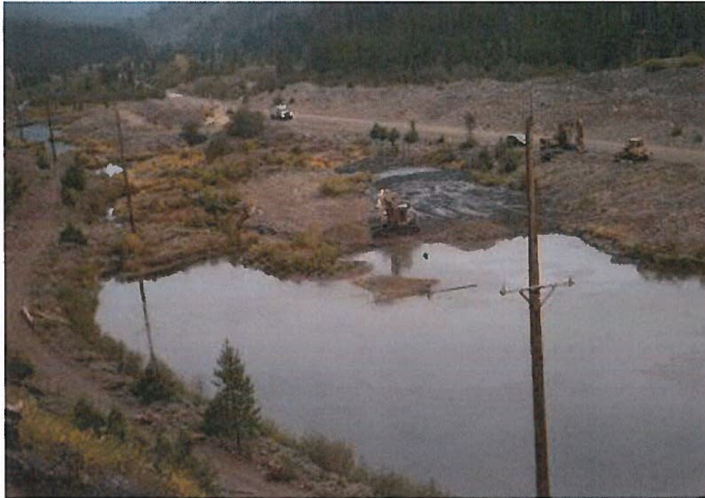
Figure 14. Removing tailings piles adjacent to and through the pond series to create a flood-plain and placing the material into the ponds to create a stream channel (middle camera photo point 24 September 2012).
