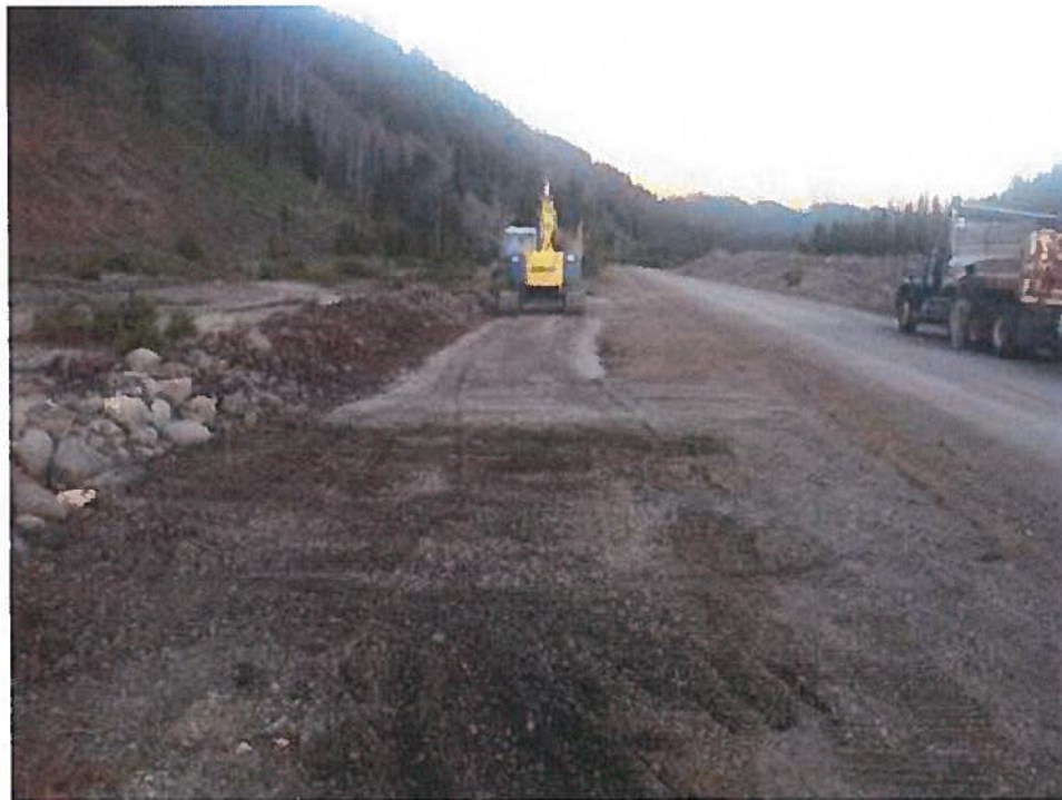
Figure 23. Building the parking area along the Pond Series 2 Side Channel project area in preparation for installation of interpretative signs.
