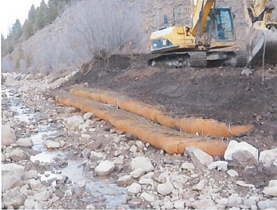
Figure 6. Removing a 36-inch corrugated metal pipe (CMP) culvert and associated fill and constructing a roughened channel (rock) upstream of, though, and downstream of the existing culvert embankment.
