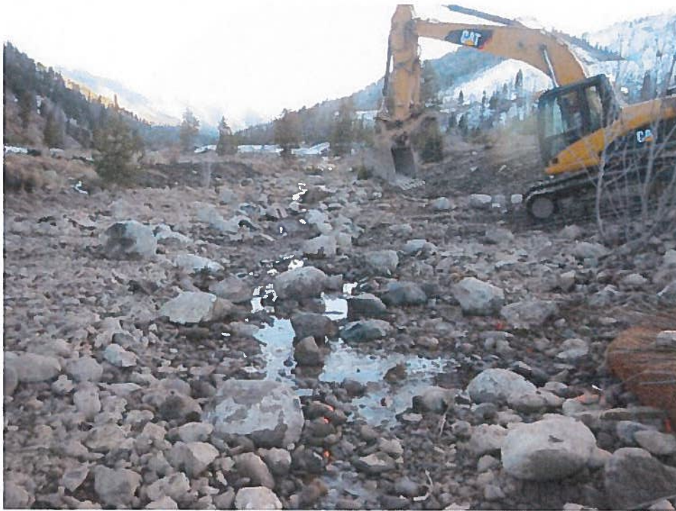
Figure 8. Placing rock to create habitat and stream stability.
