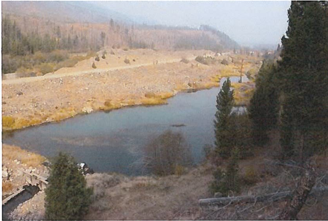
Figure 16. Removing tailings piles adjacent to and through the pond series to create a flood-plain and placing the material into the ponds to create a stream channel (lower camera photo point 22 September 2012).
