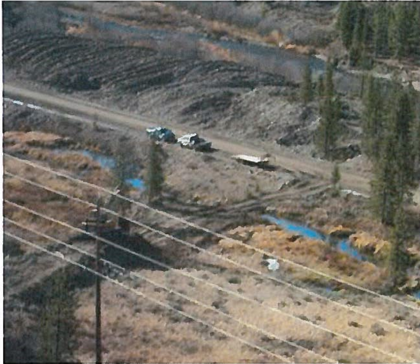
Figure 10. Removing an old road embankment across a floodplain.
