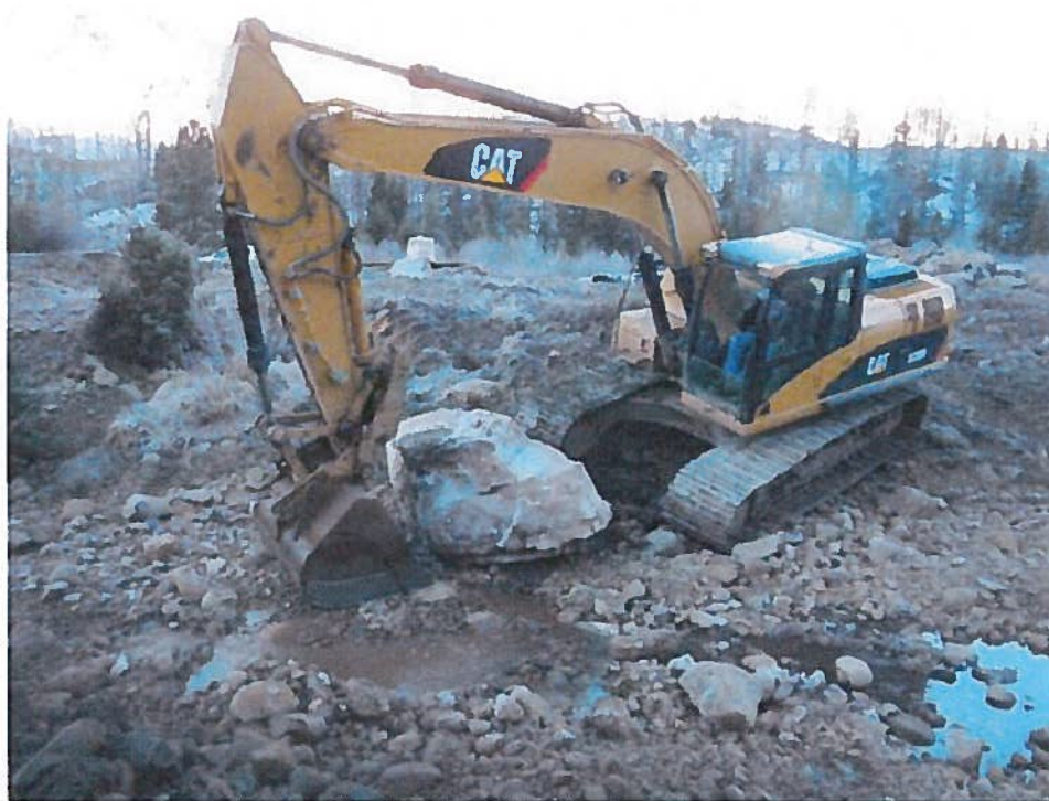
Figure 7. Placing rock to create habitat and stream stability.
