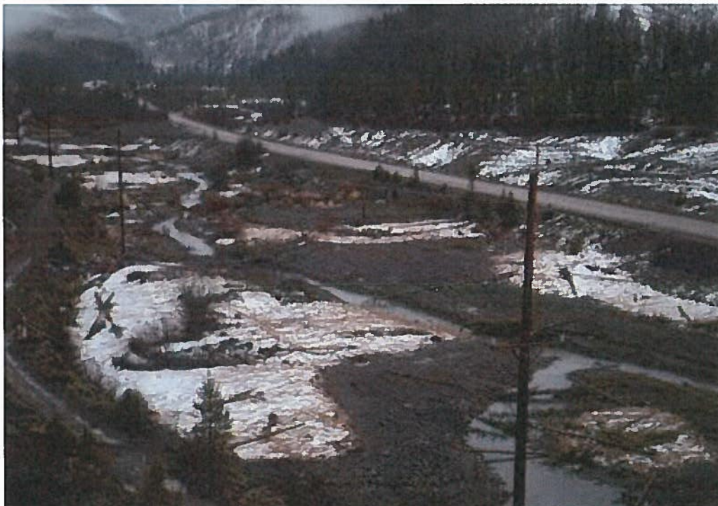
Figure 15. Removing tailings piles adjacent to and through the pond series to create a flood-plain and placing the material into the ponds to create a stream channel (middle camera photo point 20 November 2012).
