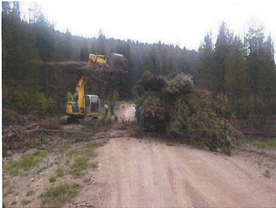
Figure 24. Trees the Forest Service cut during the 2012 Halstead Fire that were hauled to a staging area during the spring of 2013.
