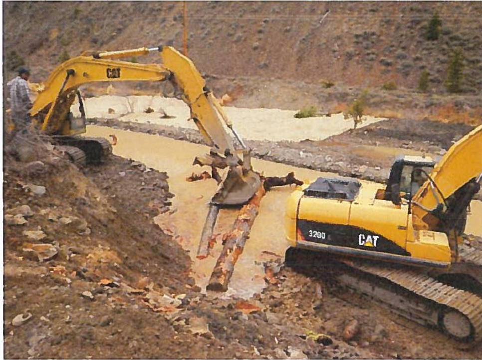
Figure 4. Placing wood habitat structures.
