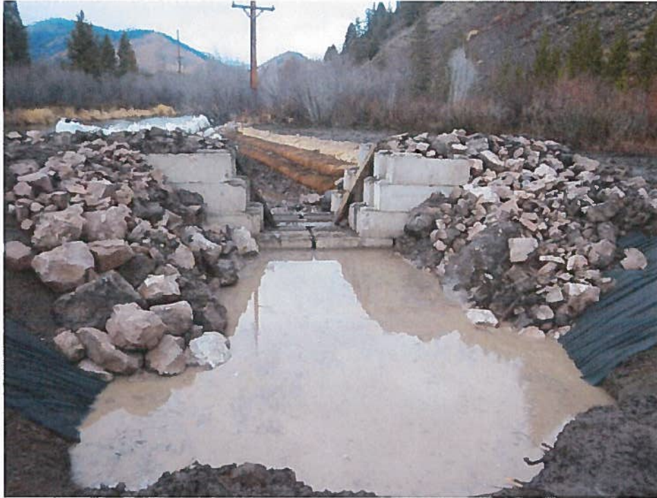
Figure 2. Constructing an inlet channel and off-channel inlet control structure (sheet pile).
