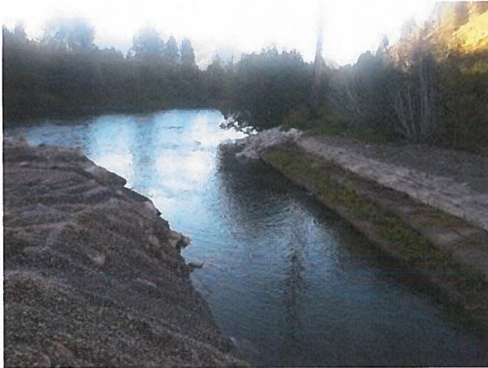
Figure 22. Yankee Fork Pond Series 3 inflow with coffer dam removed (June 2013).
