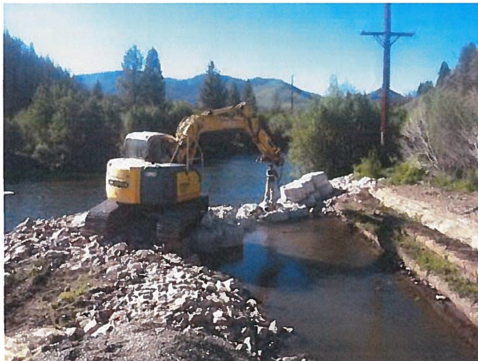
Figure 21. Removing the coffer dam after high spring flow receded (June 2013).
