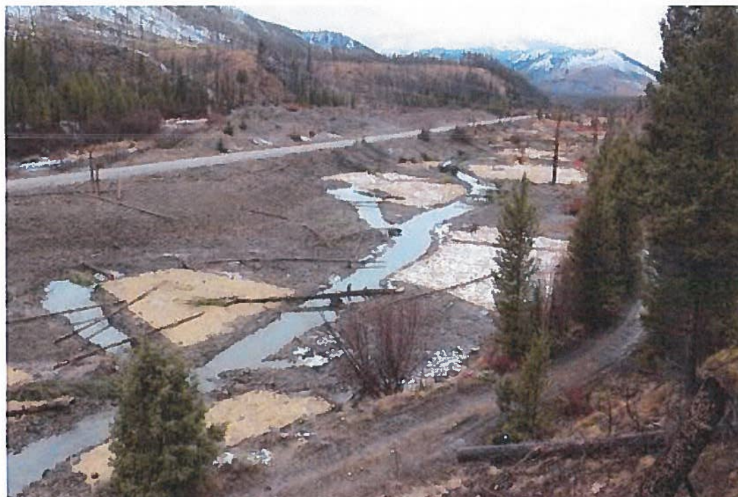
Figure 17. Removing tailings piles adjacent to and through the pond series to create a flood-plain and placing the material into the ponds to create a stream channel (Lower camera photo point 20 November 2012).
