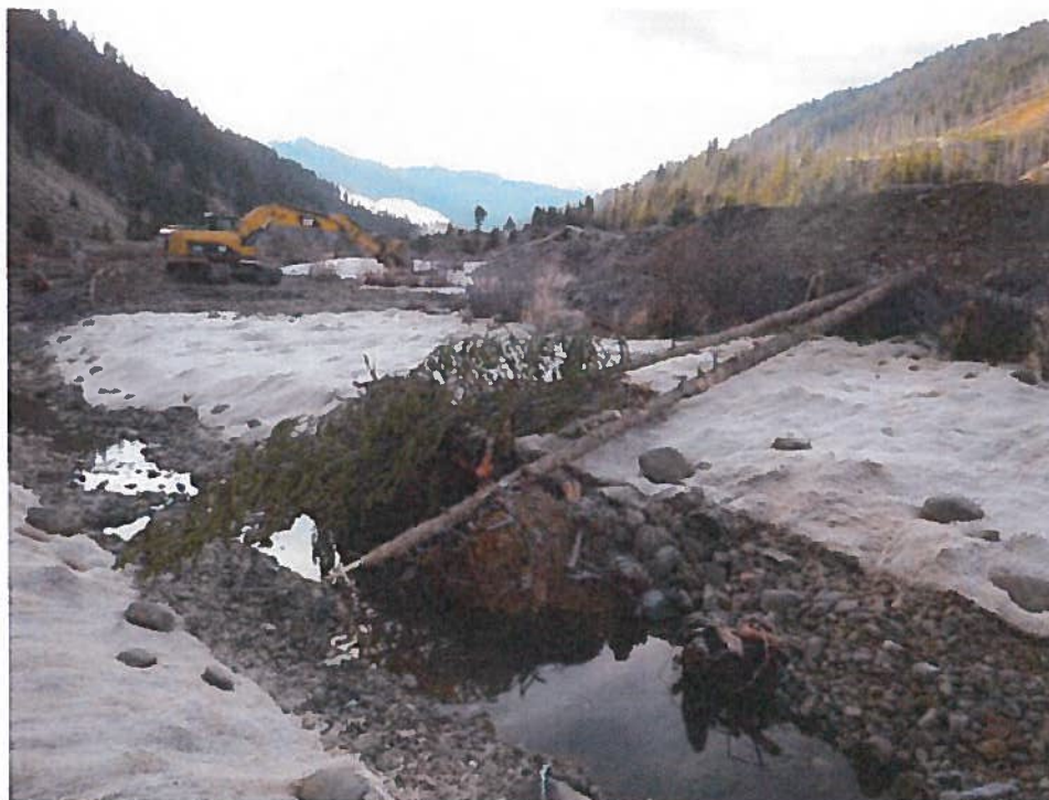
Figure 3. Placing wood habitat structures.
