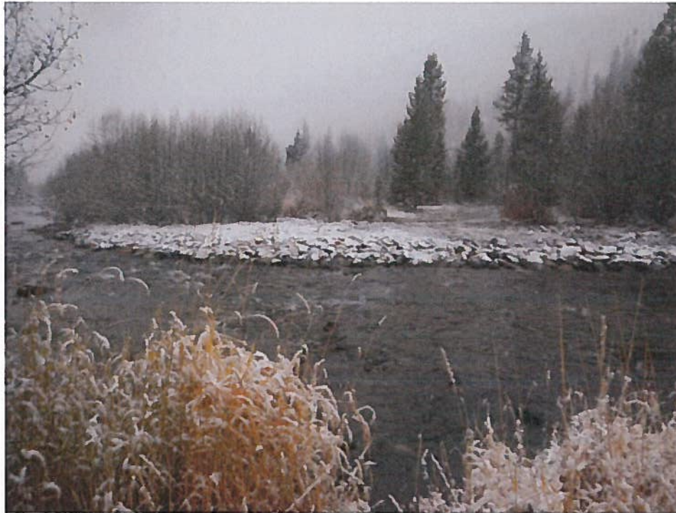
Figure 18. Creation of a point-bar to aid in formation of a pool at the outflow of Pond Series 3.
