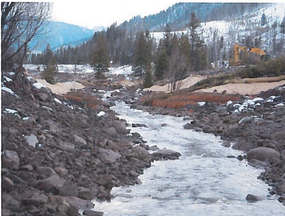
Figure 9. Roughened channel for inflow stability.
