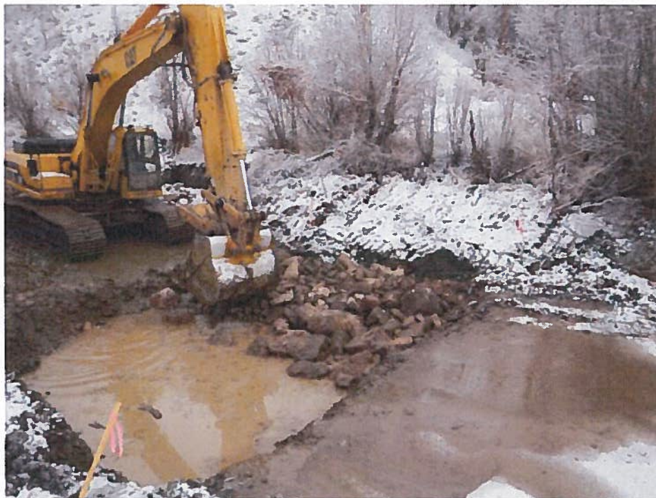
Figure 5. Installing rock weir structures for stabilization and complexity.
