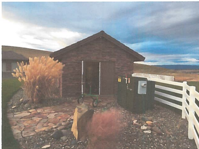
COMPLETED WELL HOUSE
