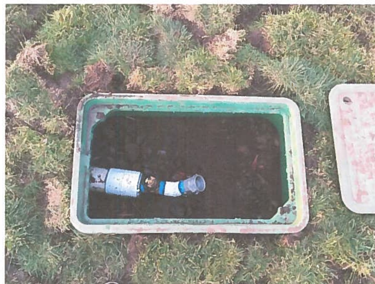
2-INCH CONNECTION FOR IRRIGATION
