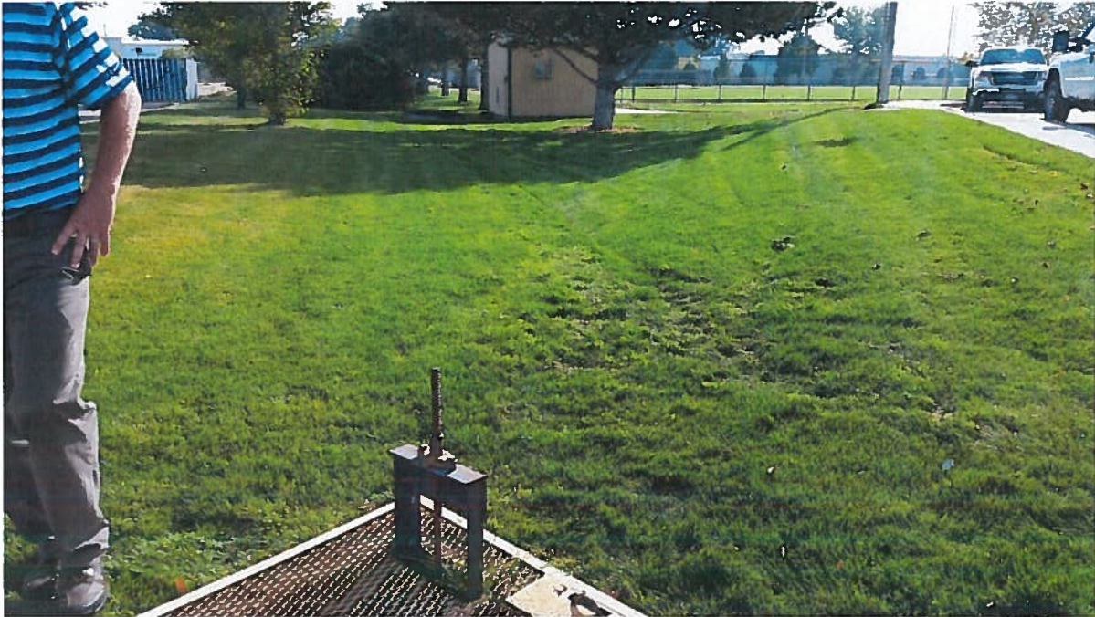
Photo 5: Looking east from the NMID delivery box towards the booster station and vault.
