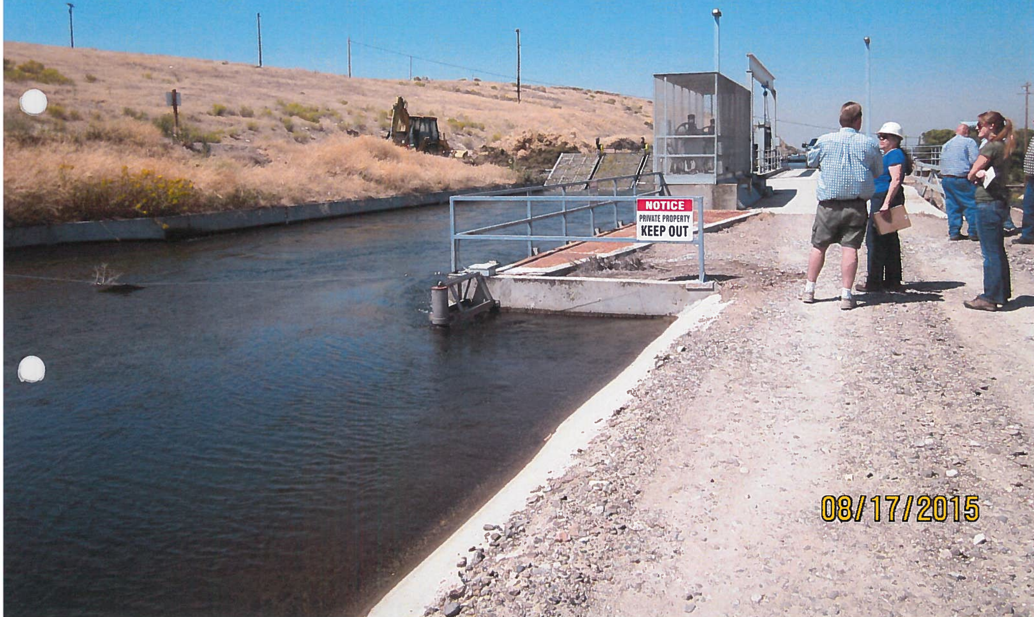
WR# 63-9206 view of the re-diversion works from the Mora canal (east) side
