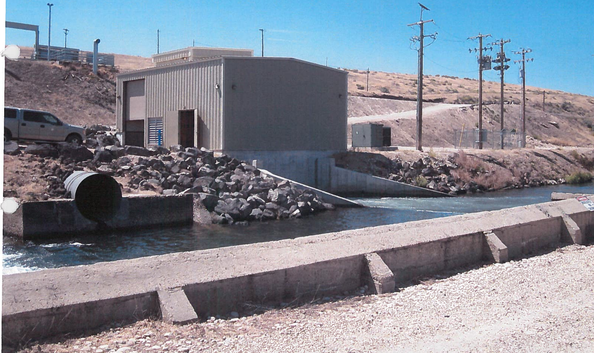
WR# 63-9206 view showing the turbine discharge
