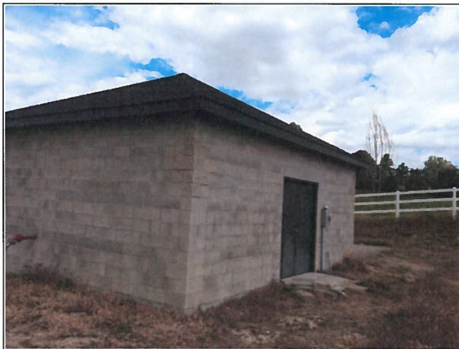
Pump House: T2N, R3W, S6, NWSE (Lot 11, Block 2)
