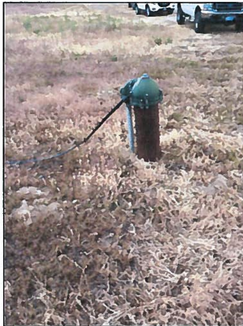
POD (Well 2): T2N R3W, S6 NWSE (Lot 11, Block 2)
