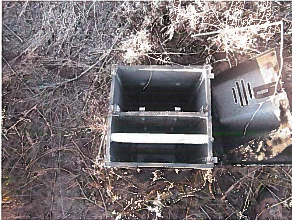
Figure 4: View inside level control apparatus-water rises up to orifice at preset height, excess flows through, cascades into outlet pipe and out to stream channel
