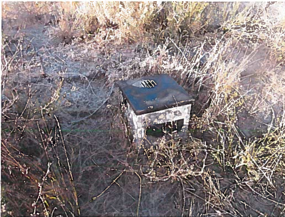
Figure 3: Access to level control structure
