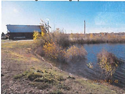
Irrigation storage pond 1 and pump house.
