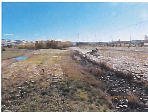
Gravel bottom trench discharging water from storm water detention pond 1 to storm water detention pond 2. Water flows towards bottom of photo.
