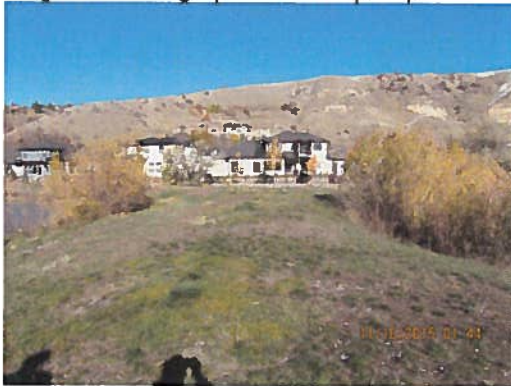
Earthen levee/berm separating irrigation storage pond 1 from storm water detention pond 1.
