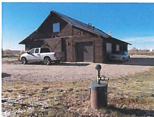
Pump house / maintenance storage at SE corner of irrigation storage pond 1. Note ground water well which pumps water into the pump house vault and irrigation pond 1. Well tag number D0064422.
