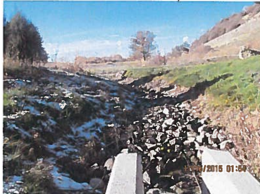
Outlet from storm water detention pond 2 flowing into ditch which ultimately discharges into the Boise River.
