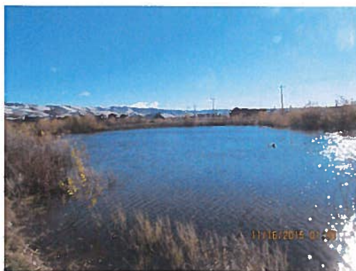
Storm water detention pond 1.
