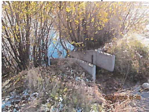
Discharge point from storm water detention pond 1 draining into storm water detention pond 2. Water flows from left to right.
