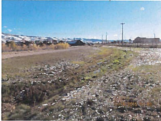
Grassy swale that delivers storm runoff from the subdivision to storm water detention pond 1.
