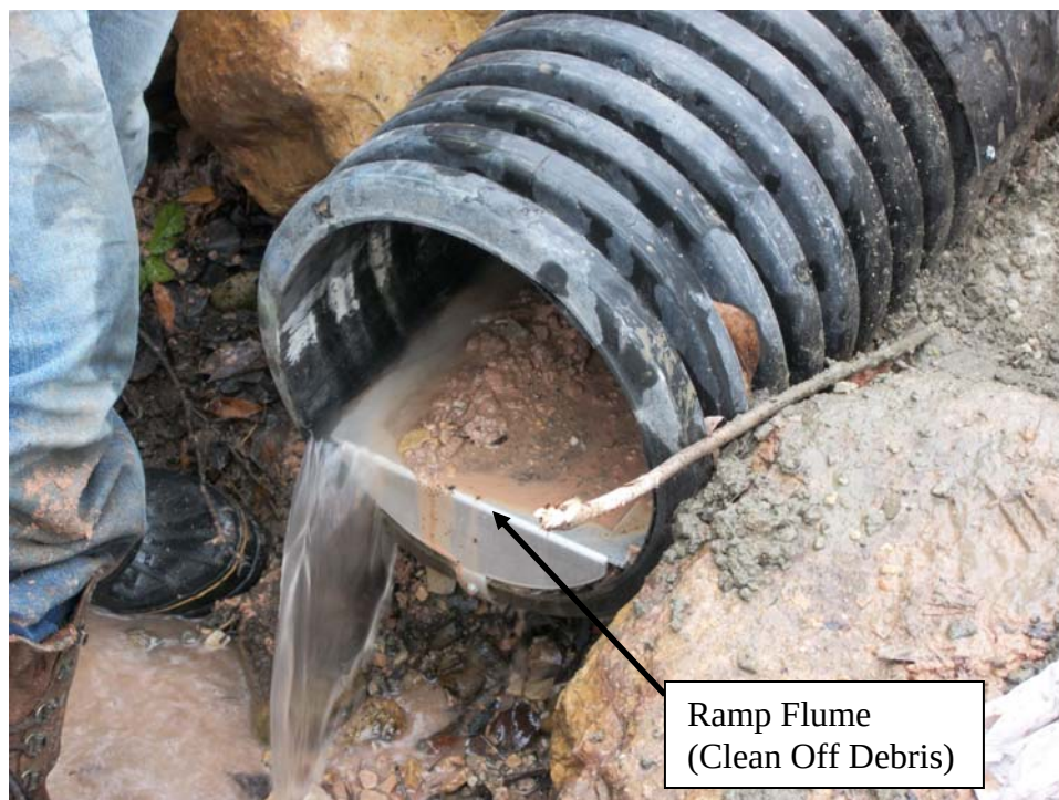
Photo 2 – Bypass Pipe Flume
