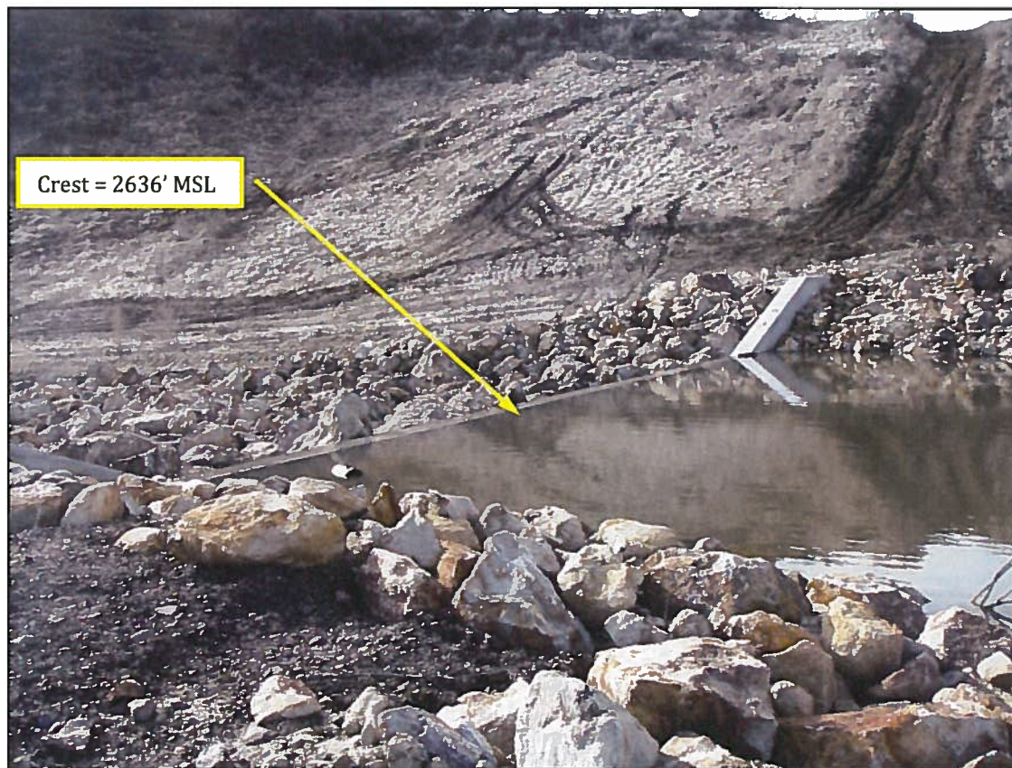
Photo 1 – Primary overflow spillway located on the south (right) side of the Auxiliary Dike. This feature regulates the pool level associated with the larger reservoir impounded by the Main Dam and the Auxiliary Dike. Water to fill the 1859 AF reservoir is diverted from Dry Creek via a canal. As shown, the crest of the concrete weir at the Auxiliary Dike defines the maximum pool.
