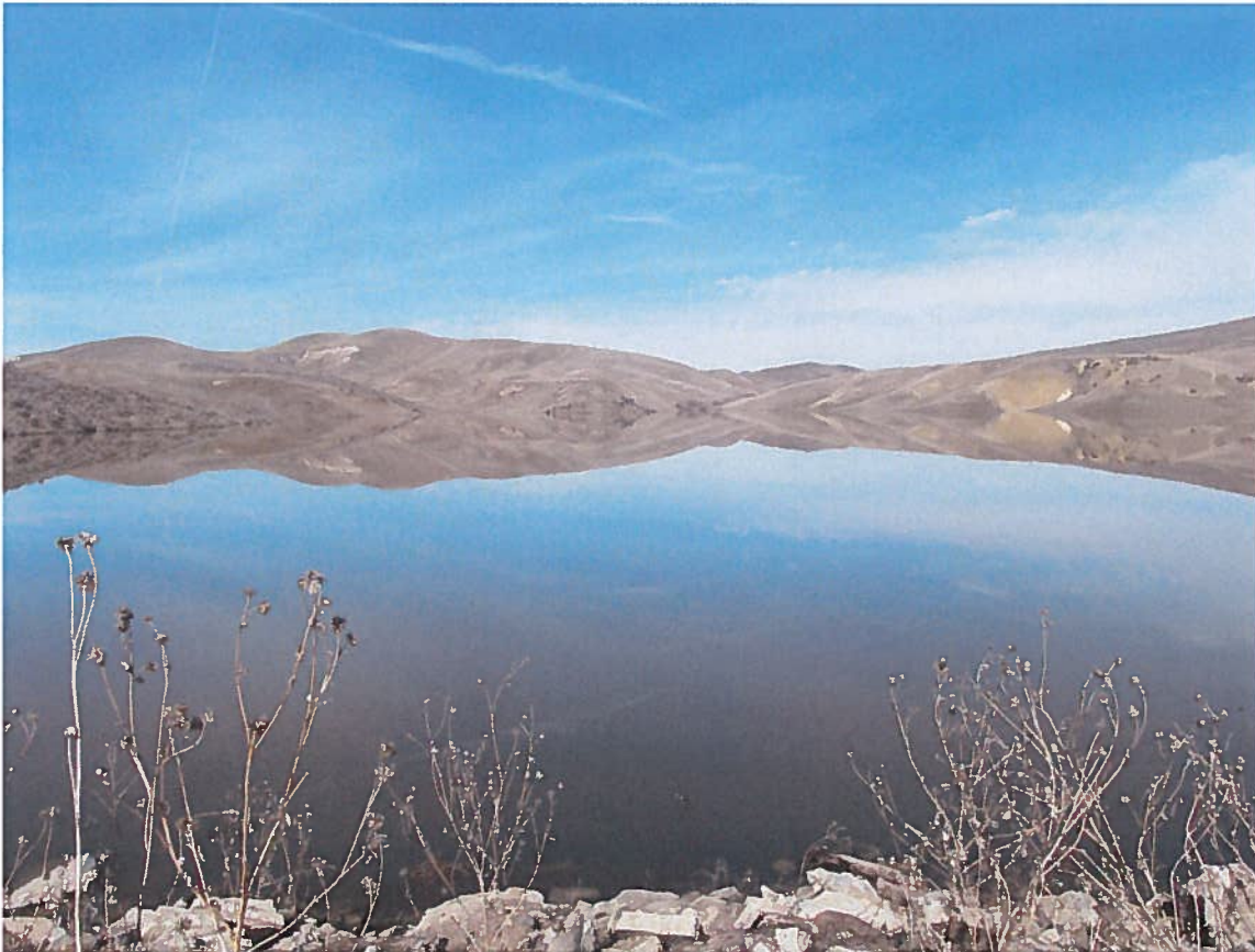
Dry Creek Reservoir was full at the time of the site visit. This was the reservoir view from the Main Dam.
