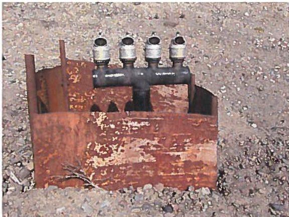
(Left) We observed the four large vents at the toe of the Main Dam. (Right) Farther down the access road, we stopped to look at the outlet valve and vent.
