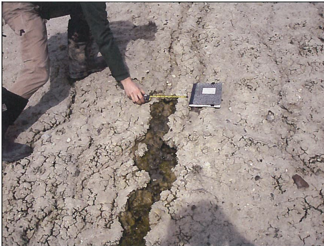
Photo 5 – Close-up showing the origin of one of the larger flowing leaks, estimated @ 2 gpm.
