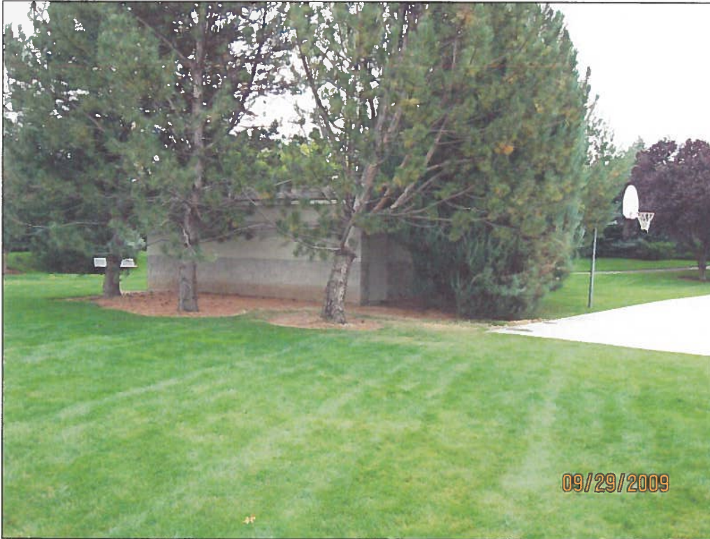
Figure 1: Well #1 pump house.
