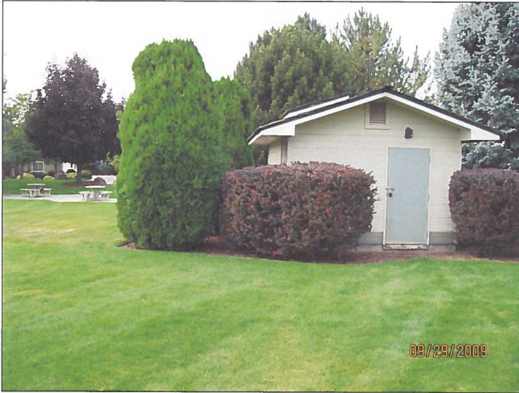
Figure 5: Well #2 pump house.
