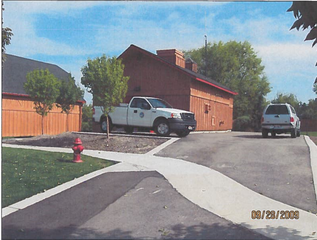
Figure 9: Well #3 pump house.
