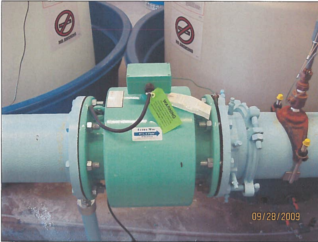
Figure 13: Well #3 McCrometer UltraMag flowmeter.
