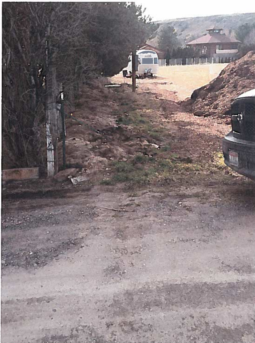
Above: View looking south towards the applicant's POU. Evidence of trench for buried pipe across the road and onto applicant's property.
