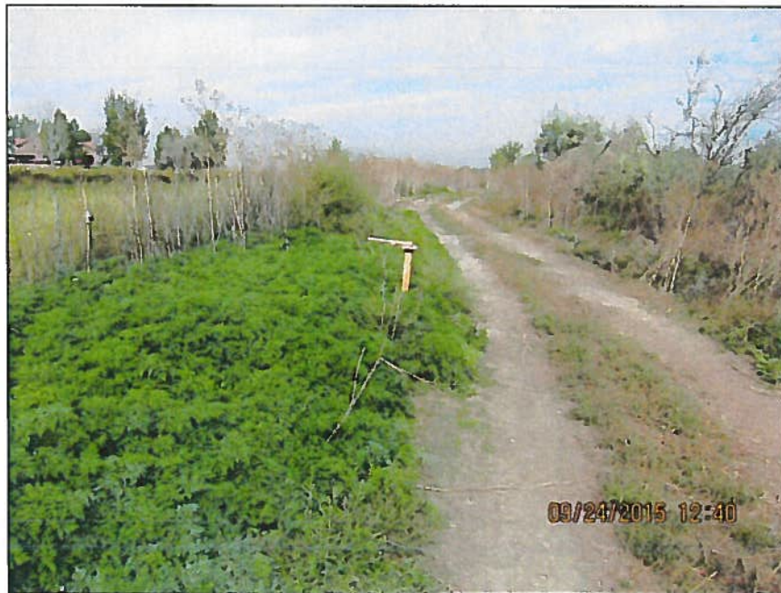
Figure 4: Valve for turning water into place of use "D" (on photo right).
