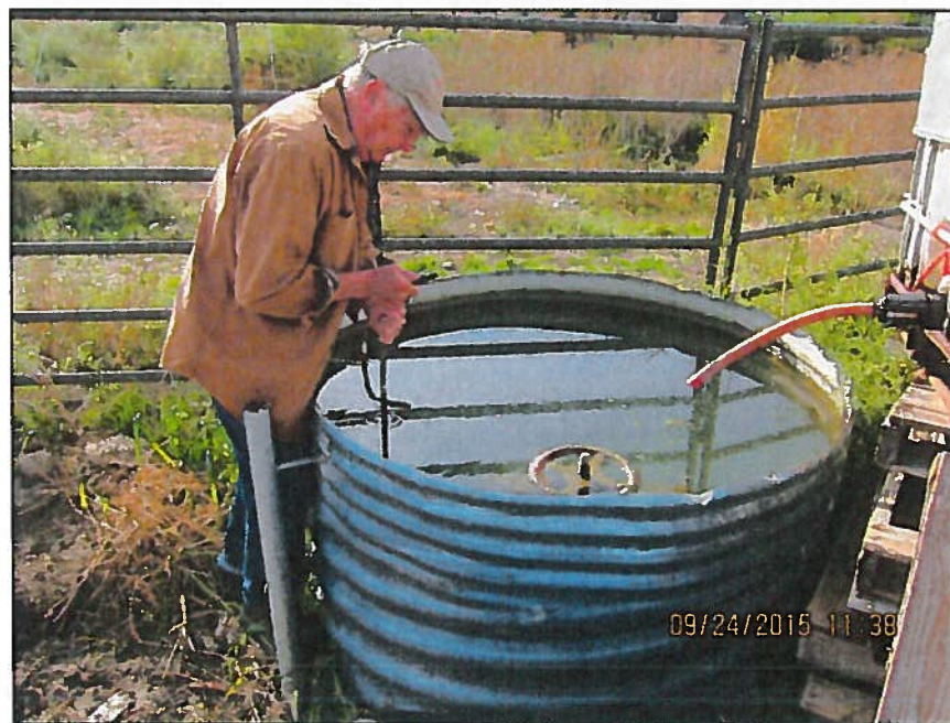
Figure 2: Check and control structure receives water piped from point of diversion.
