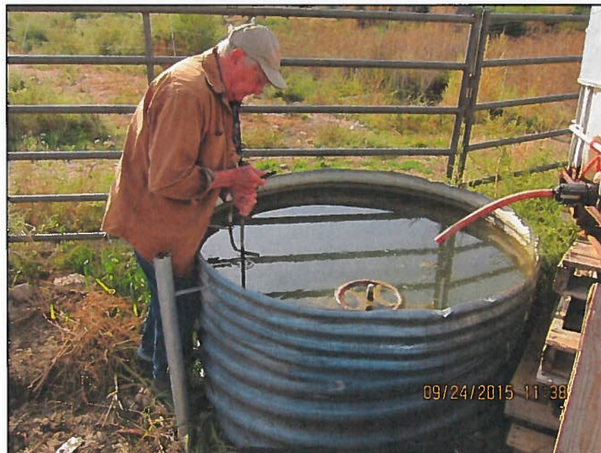
Figure 2: Check and control structure receives water piped from point of diversion.
