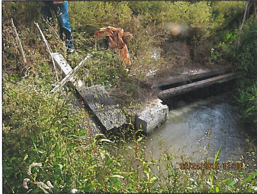
Figure 1: Point of diversion is on left at slide gate lying on ground. Flow on right enters Ross East End Drain.
