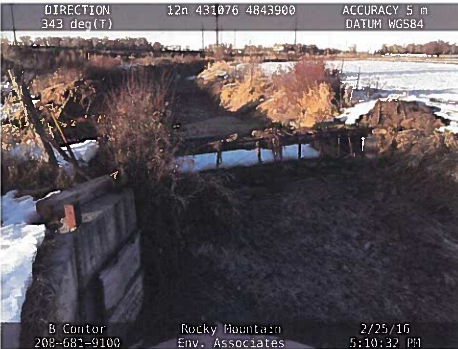
Figure 16. Lateral headgate from Liberty Park Canal, discharging to the west (photo left).
