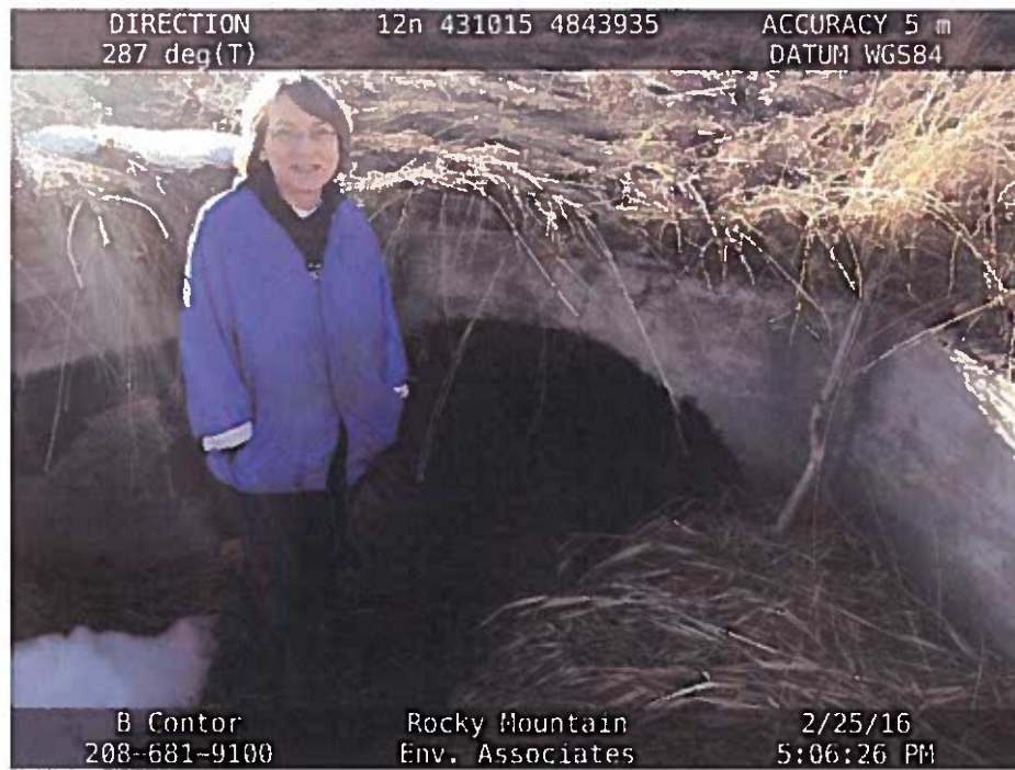
Figure 17. Lateral culvert under US Highway 20.
