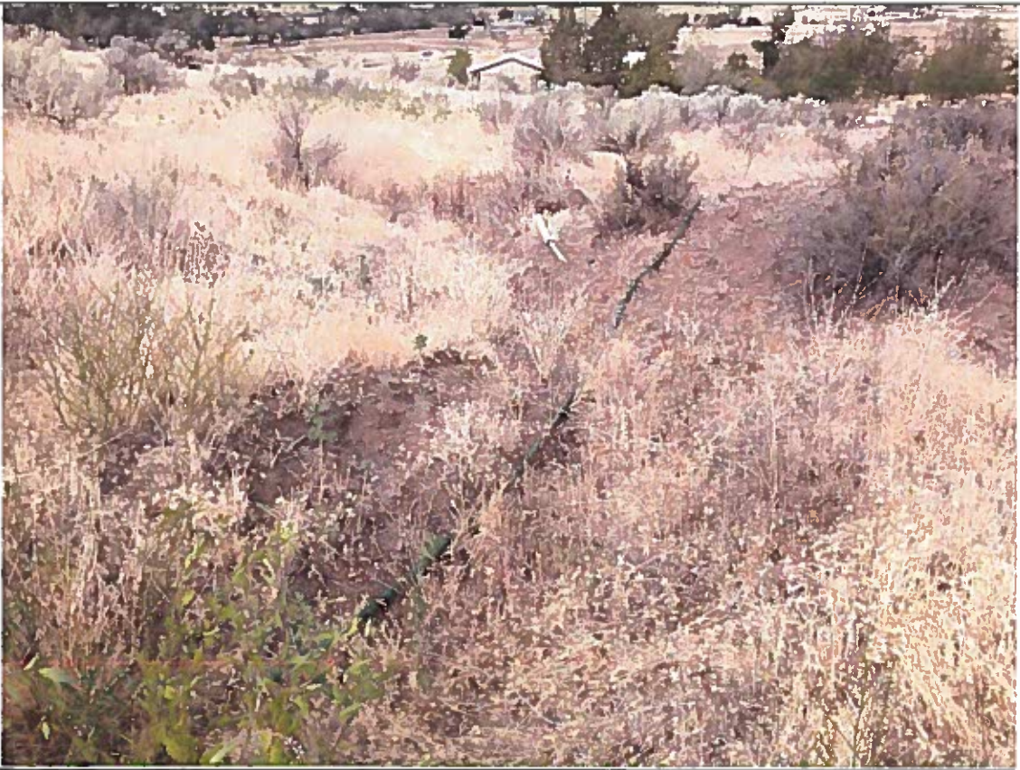
Standing at spring box, looking west towards house (POU). 2" PVC diverts to domestic tank.
