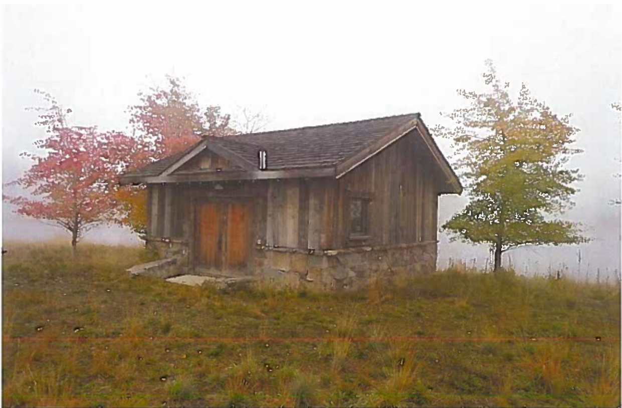
View of the irrigation pump house located between the large and small storage ponds. Water is pumped from Well No.1 to the pump house for the pressurized irrigation system.
