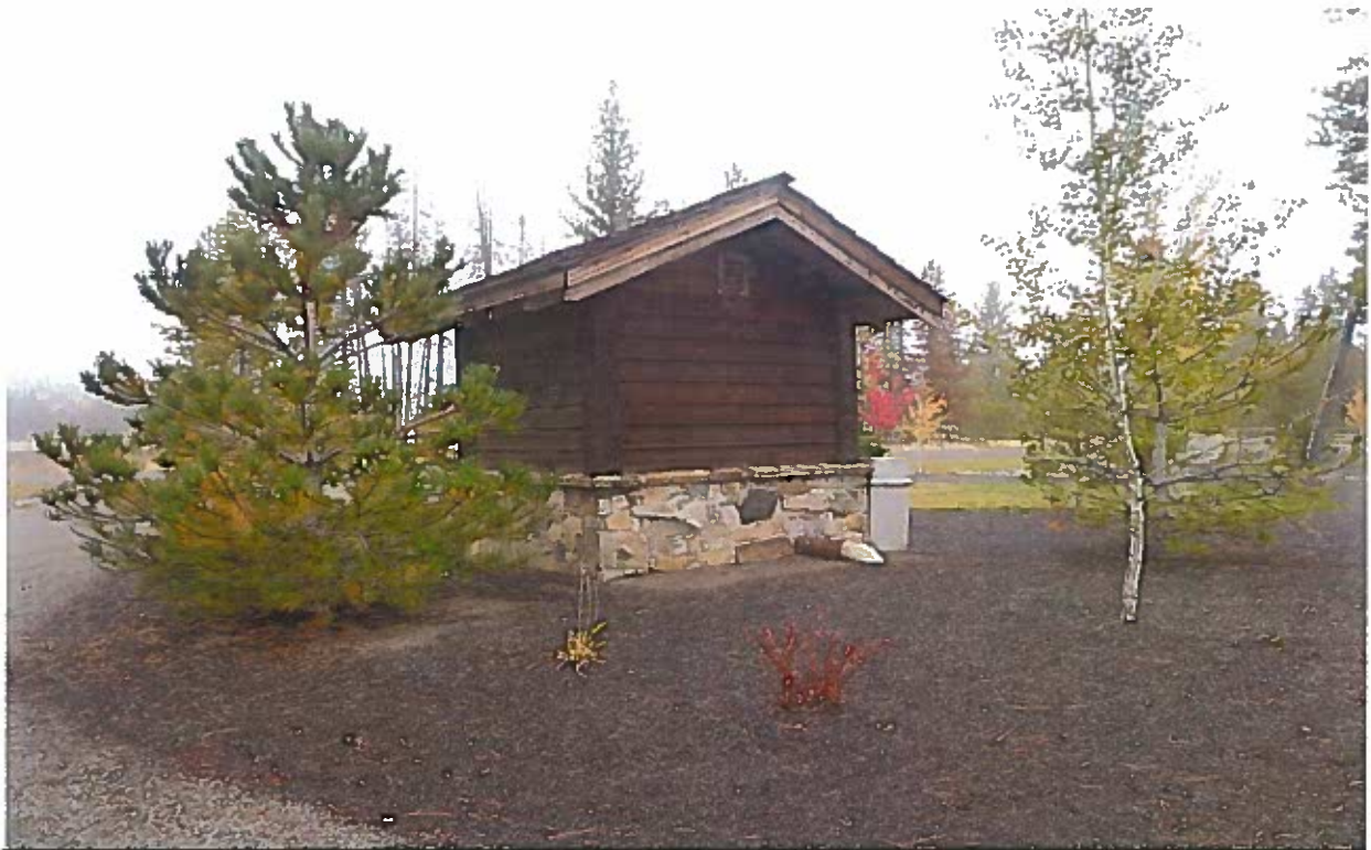
Point of Diversion: View northwesterly of well/pump house for Well No.2. Water is pumped from Well No.2 to the distribution main lines in the well/pump house which houses Well No.1. Well No.2 is primarily used as a backup to Well No.1.
