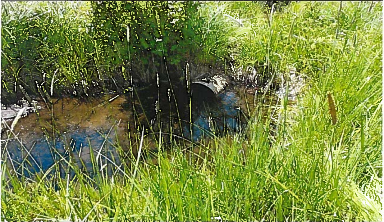
Point of Diversion: View southerly of a culvert pipe discharging water from an Unnamed Stream to the recreation and aesthetic storage pond inlet channel.
