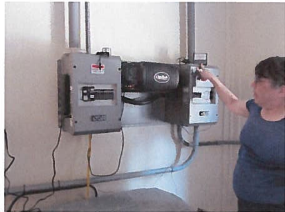
Left: We followed Mrs. Linhart along the buried power service, to the power room in the stables barn. Right: Michele points to the DC Amp meter above the inverter system, instructing me to get a photo.
