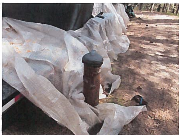
Left: The power service line from the hydropower unit was buried in a straight path uphill to the "power room." Right: The domestic well was double tagged (deepened).
