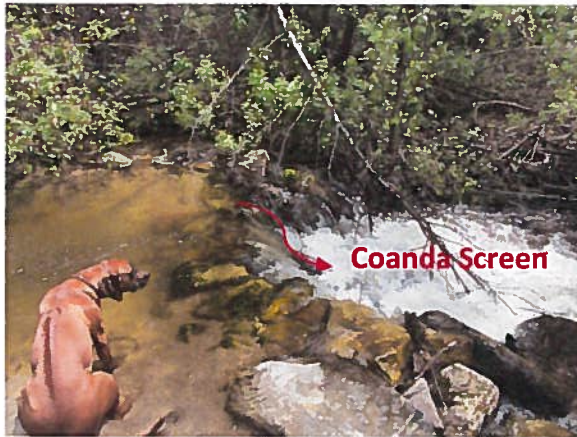
Left: The Coanda screen intake was constructed into a stream drop of approximately 3 feet. Right: The penstock runs down Yellow Pine Lane to the Stream Engine shelter.
