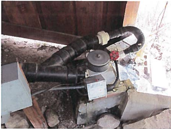
Left: The Stream Engine is a turbine-generator combination unit. It supplies the great majority for the Linharts. Right: We followed the turbine discharge back to Middle Fork Thorn Creek (source).
