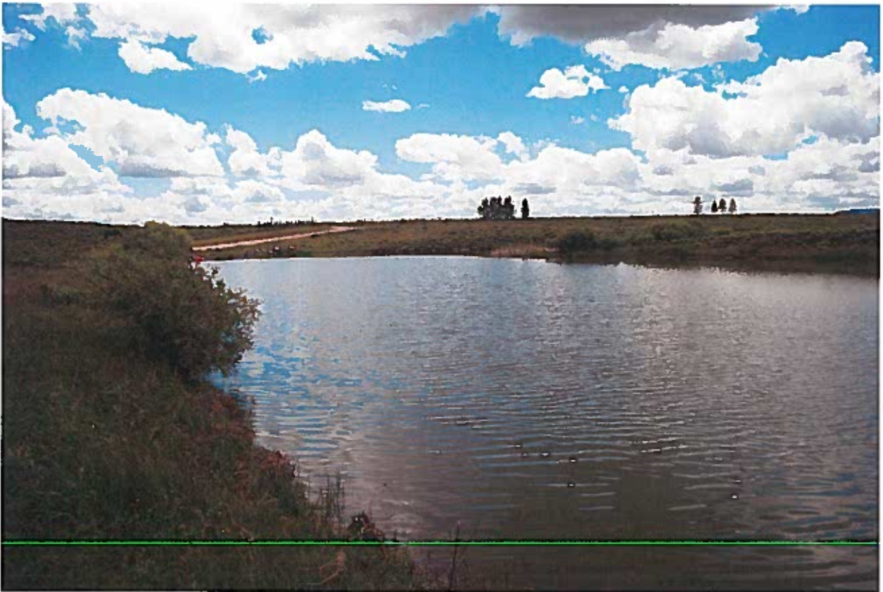
Looking south towards Pond 4 spillway
