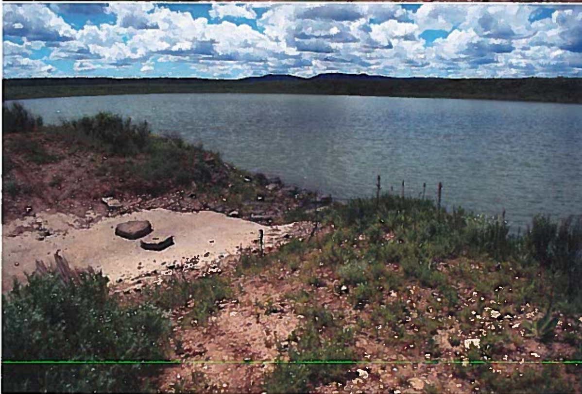
Outflow to Pond 4 at dam
