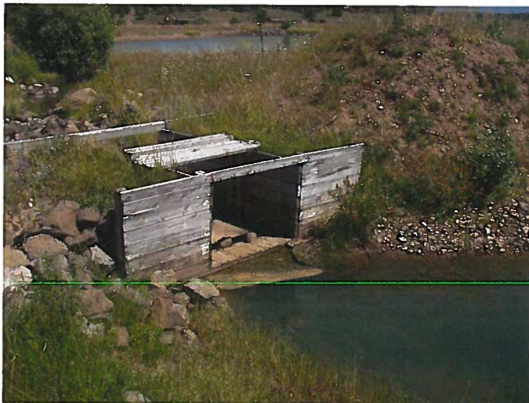
Below: Outlet at left side of Dam.
