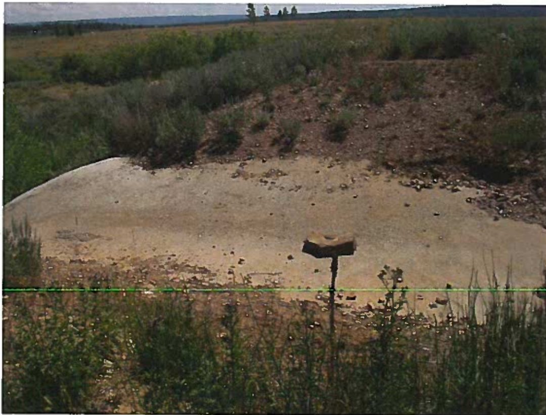
Below: Emergency spillway at center of Dam.
