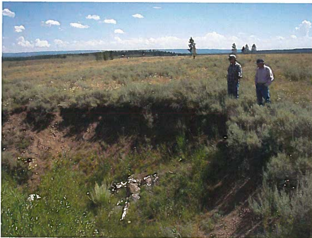
Above: Historic headcut on right abutment. Right abutment is lower than the crest of the dam.
