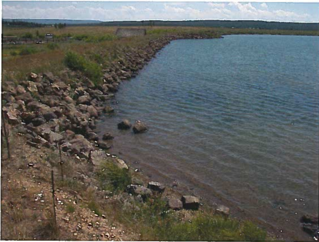
Above: Upstream slope of Dam with new rip rap from left abutment.
