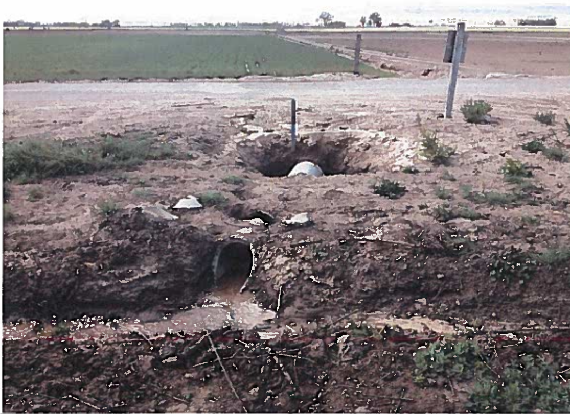
SW corner of property shows waste water passes under Pear Ln. and to wastewater ditch shown across street.
