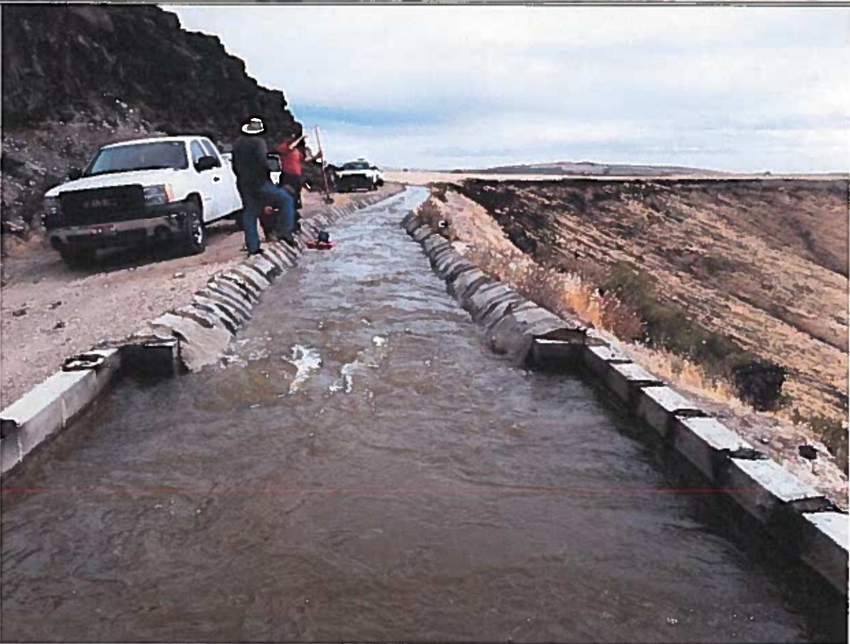
Ditch head on ridge facing NE.
