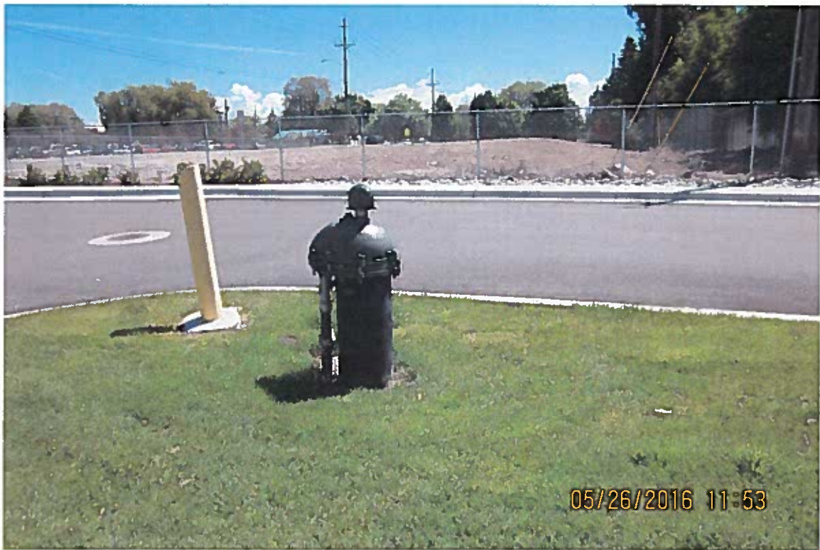
Point of Diversion
